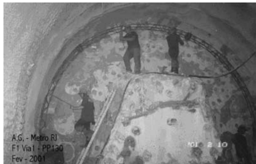
Figure 7. Septum and installation of yielding arch.
