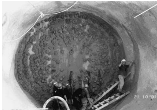
Figure 6. Tunnel face with starting drilling points.
