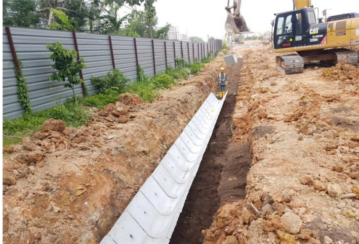
Figure 7: Laying of C7 drain
