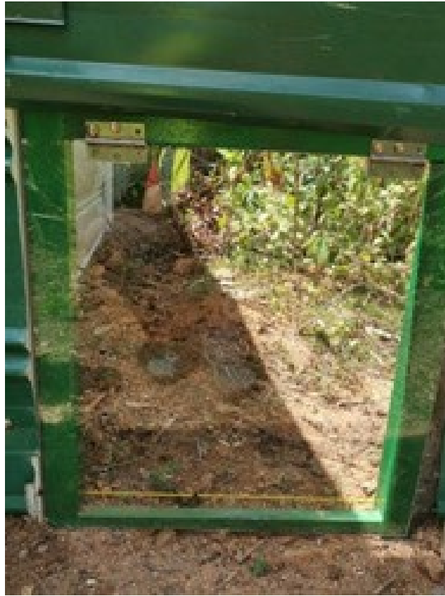
Figure 62: Example of a one-way flap door to allow fauna to exit independently
