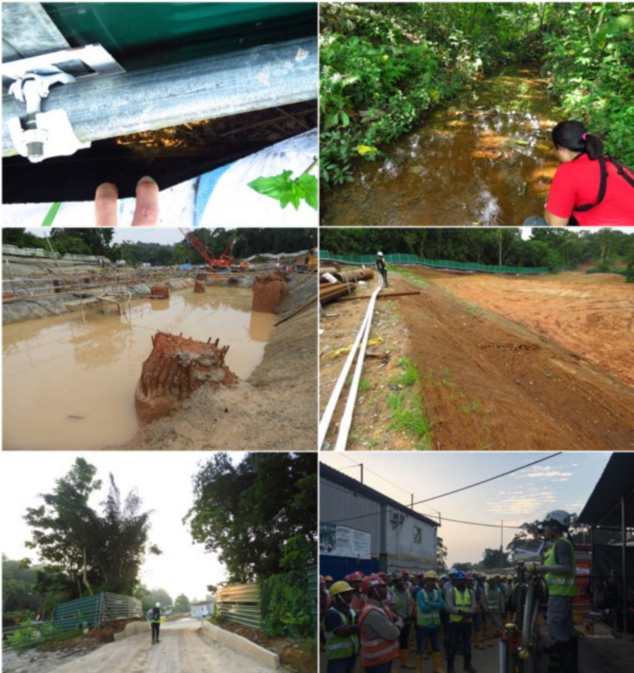
Figure 60: Photographs showing monthly fauna inspections to ensure integrity of hoarding, inspect sensitive habitats in proximity, ensure there is no trapped fauna (e.g., in ECM sedimentation ponds, erosion control blankets), and biodiversity awareness training for site personnel
