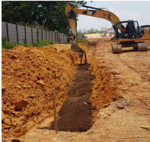
Figure 6: Laying of sand for C7 drain
