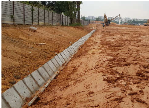
Figure 8: Compaction of slope adjacent to C7 drain
