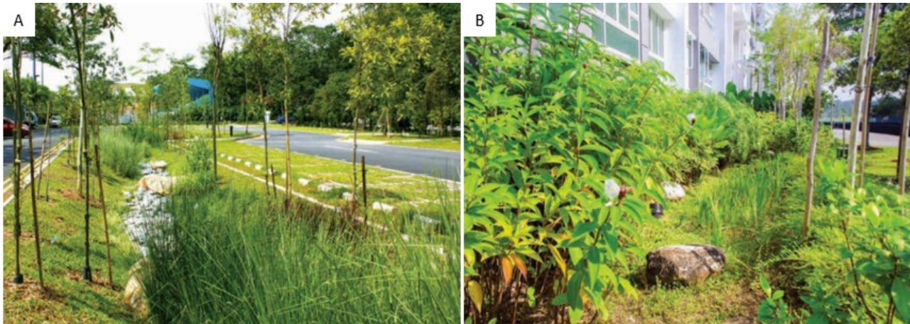
Figure 42: (A) Example of vegetated swales integrated in carpark facility; (B) Example of bio-retention basins
