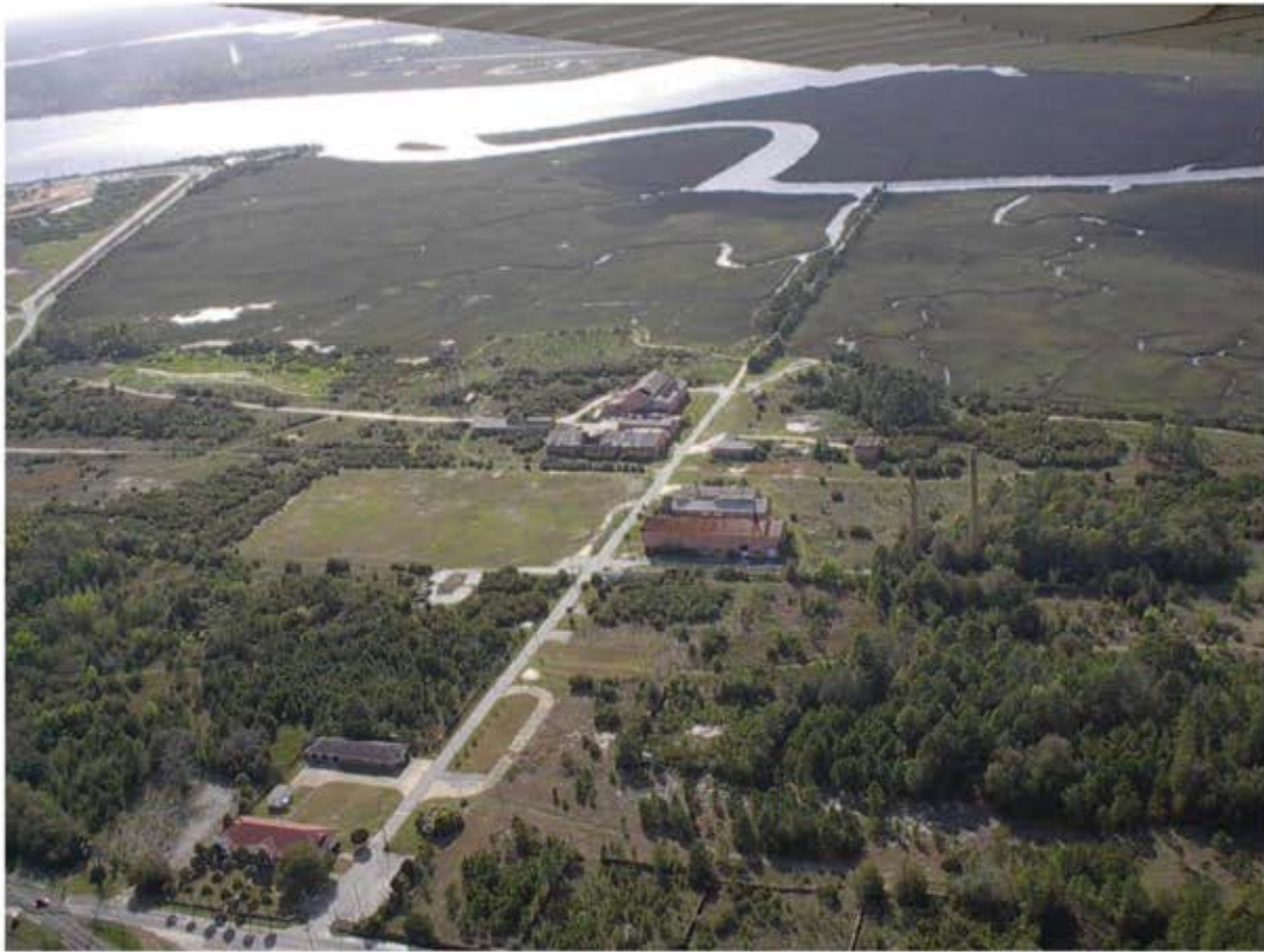
Figure A2. Site Map Showing Current Onsite Structures on Dry-land Area with Marsh in Background (March 2004)
