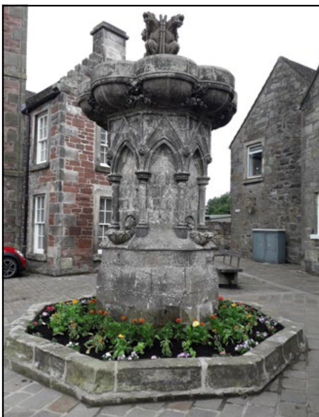
The restored Crosswell Fountain
