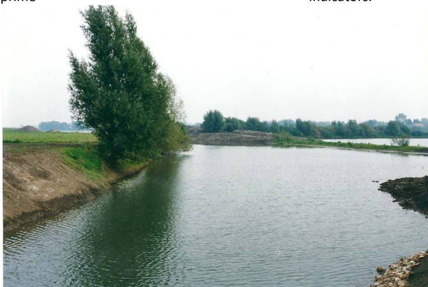
Photo 13 Newly dug side channel along the Dutch Rhine (1994)
