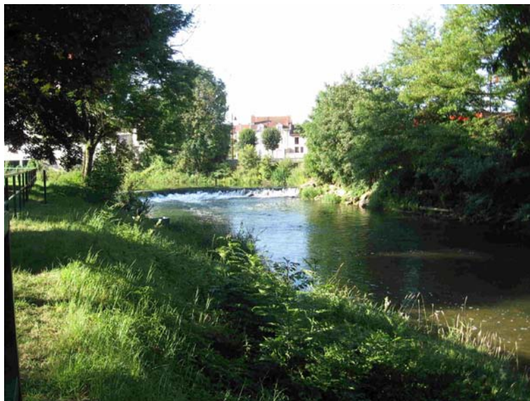
Photo 3. Example of a small dam upstream in the Marne at Froncles
