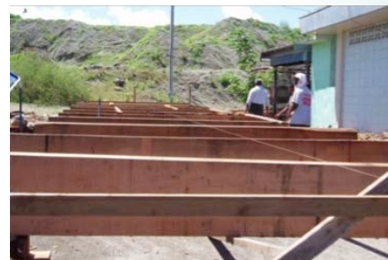
The ten sleepers (foundation beams) of Bai ra Klobak.
