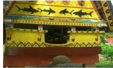
The iis (threshold) is framed on either side by doorposts called chad , and both rest on the kuoku beam.
