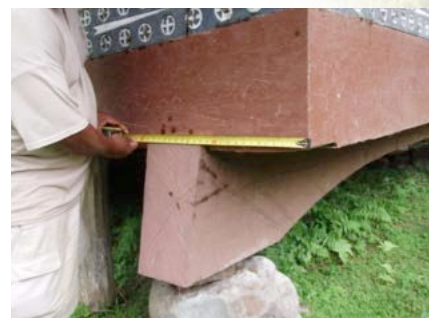
The foundation sleepers rest on top of the stone piers.
