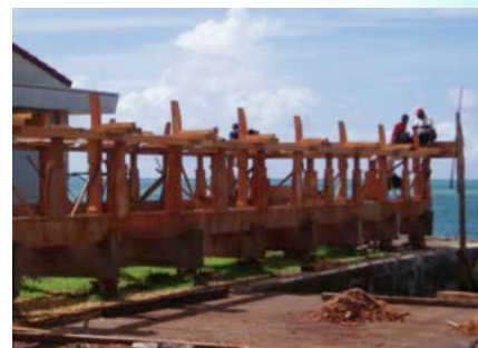
Two longitudinal uchutem beams rest on top of the ten sleepers.
