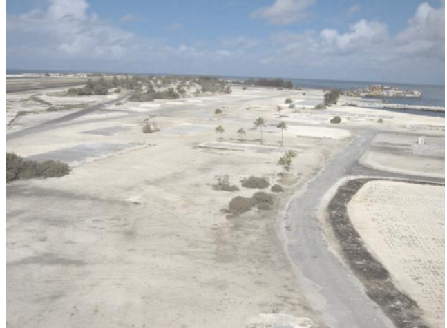
Johnston Atoll after demolition (2004)
