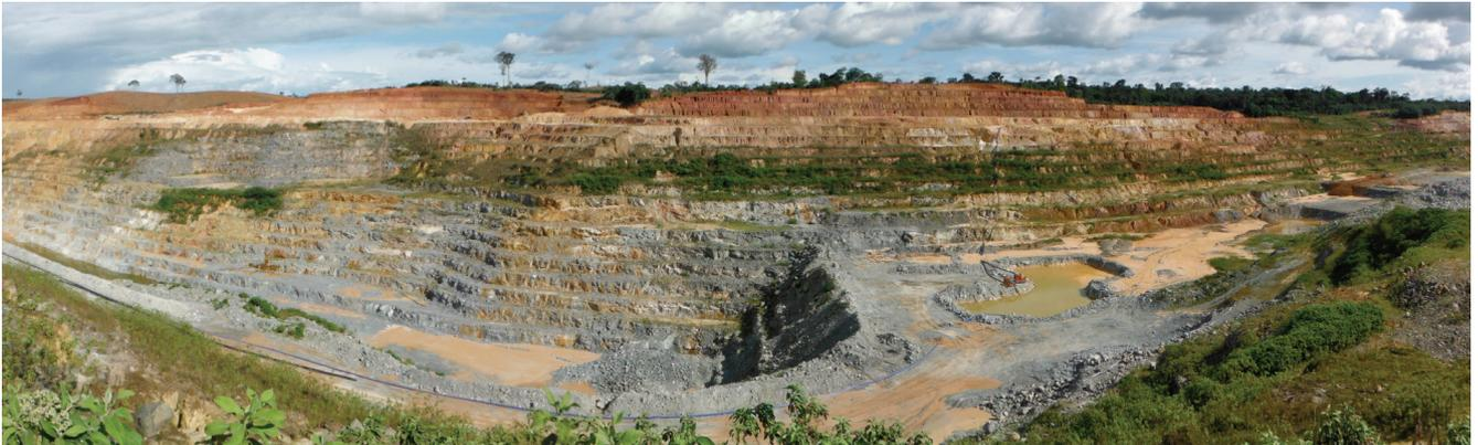
*Figure 13 – Staggered benches in Mayo Pit resulting in manageable working conditions during the wet season; and stable saprolite slopes (looking south)*
