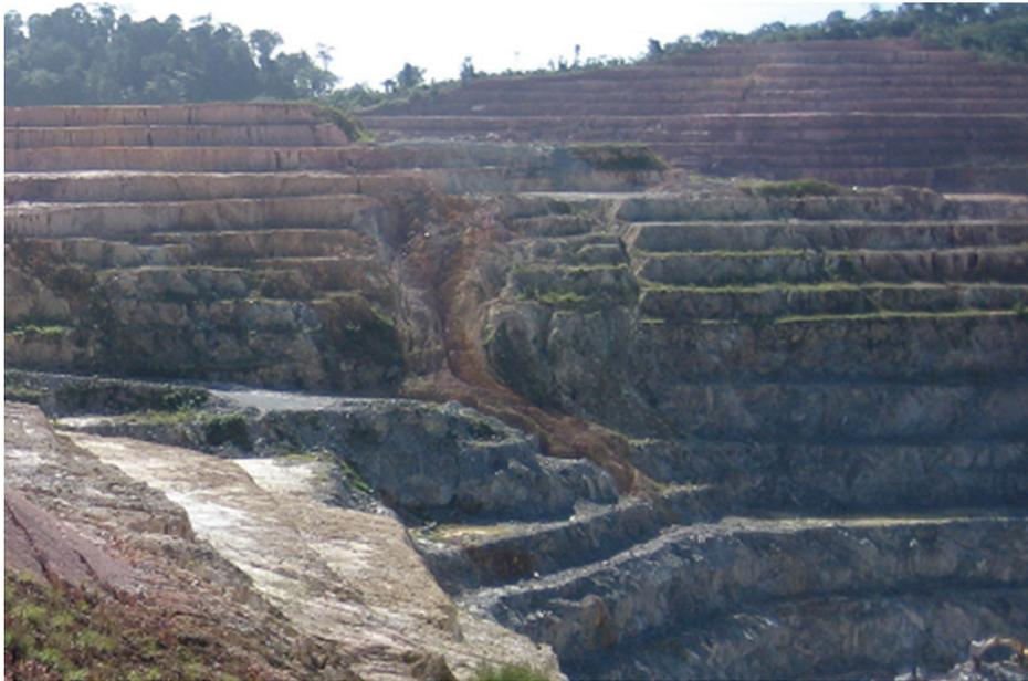
*Figure 3 – Gullying and erosion on the eastern wall of Royal Hill Pit leading to washout of material over benches below*
