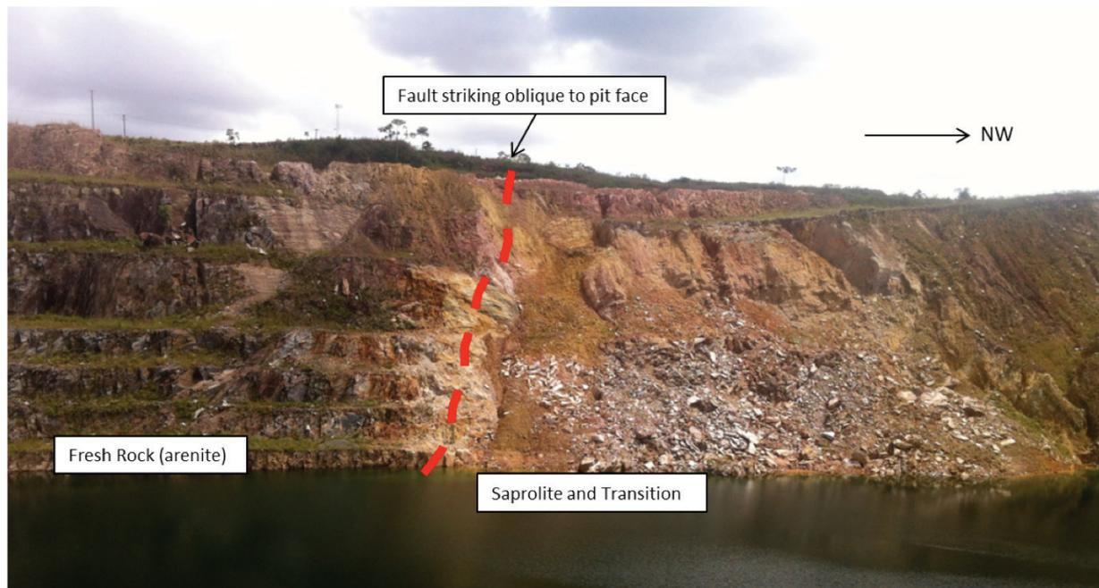
Figure 1 – Sharp contrast between fresh rock and transition due to a large fault striking oblique to the face
