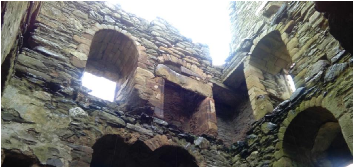
Third floor – interior arrangements to the north-east including fireplace and large mural recess at the angle.
