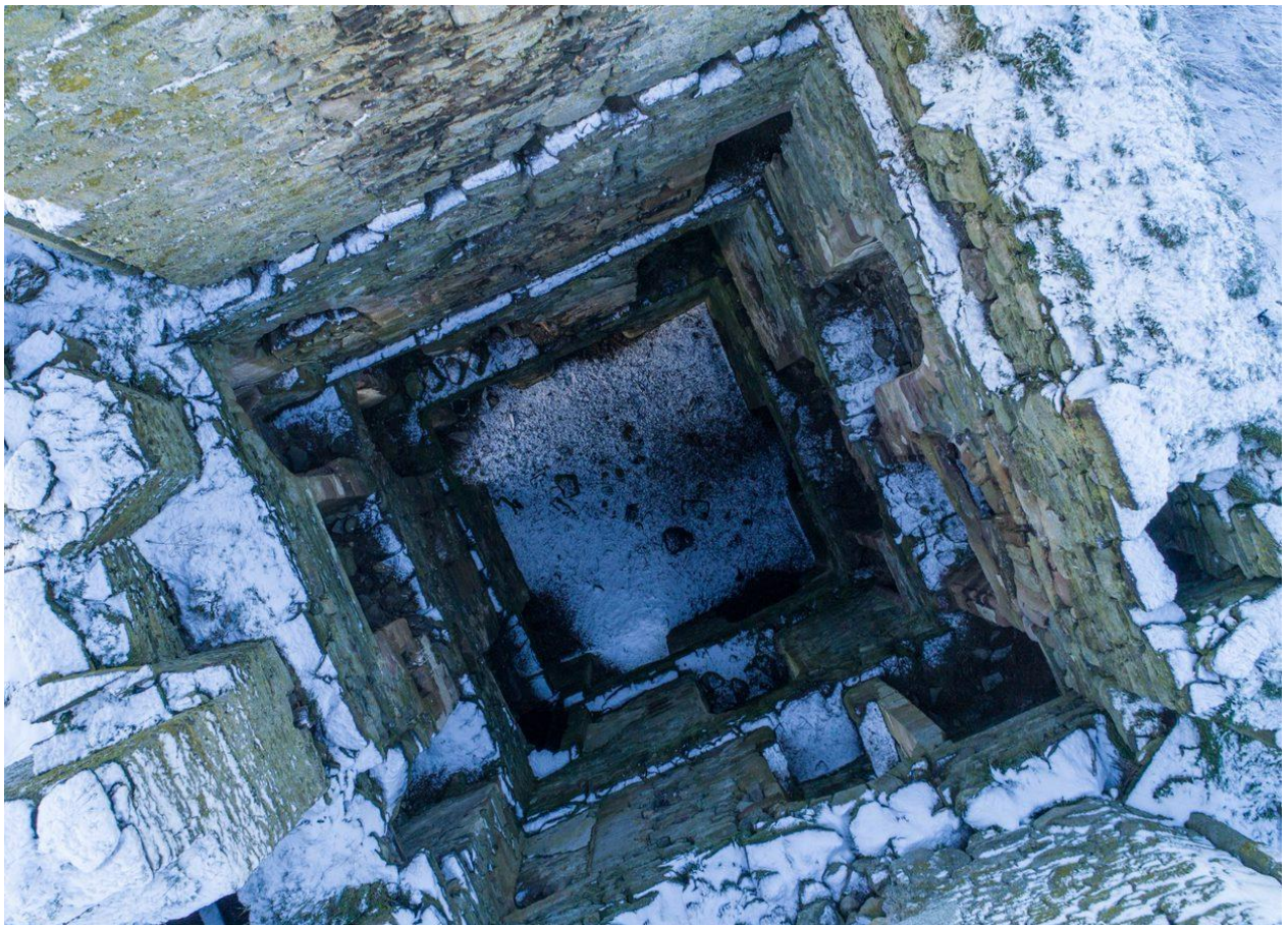
Drone shots of Fairburn Tower before restoration, in winter 2018. It stood as a completely gutted shell.
