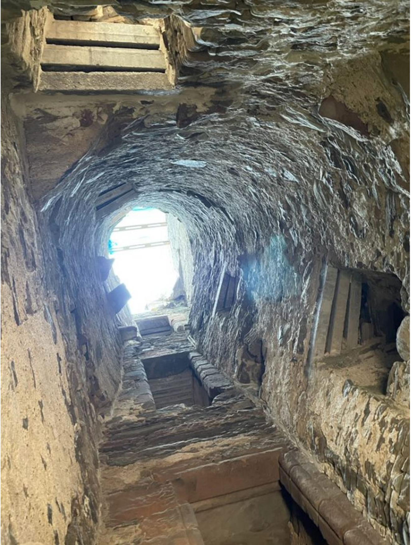
Interior of the stair tower.
