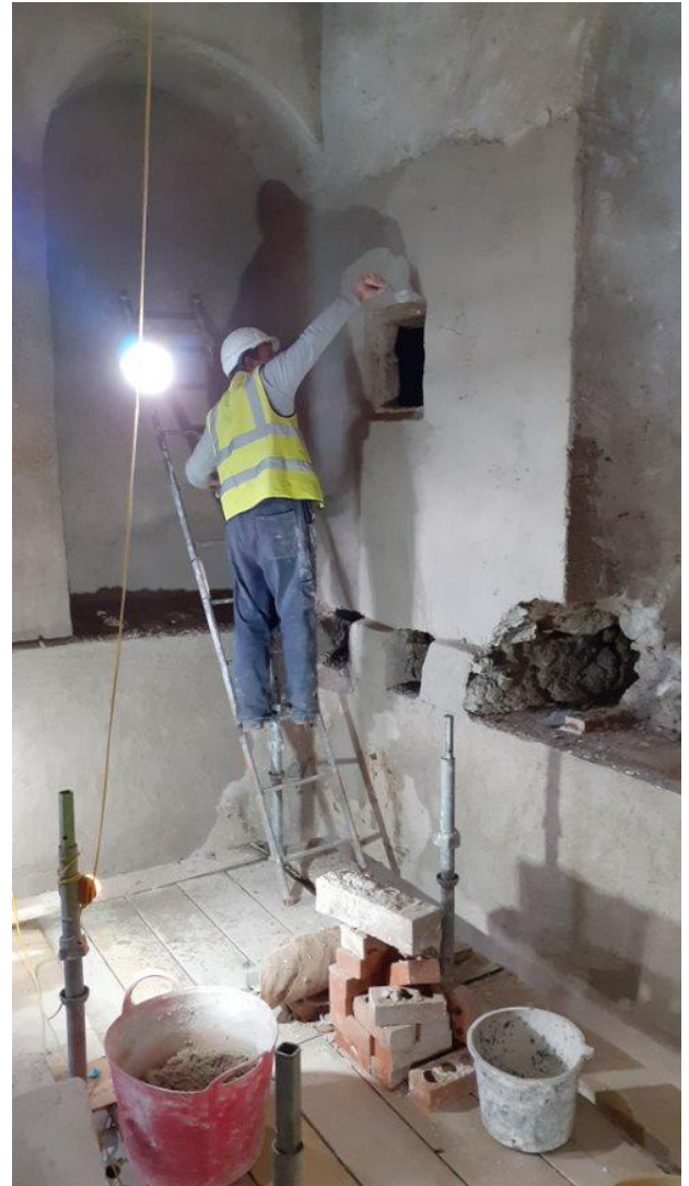
Meanwhile, with all floors reinstated, work was well underway with plastering the rooms of the tower.
