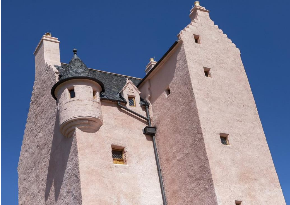
The stair turret, one of the two bartizans and the dormer with its datestone, all reconstructed along with the inhabitable top storey in 2020-22. They were originally added to the main tower c1600.
