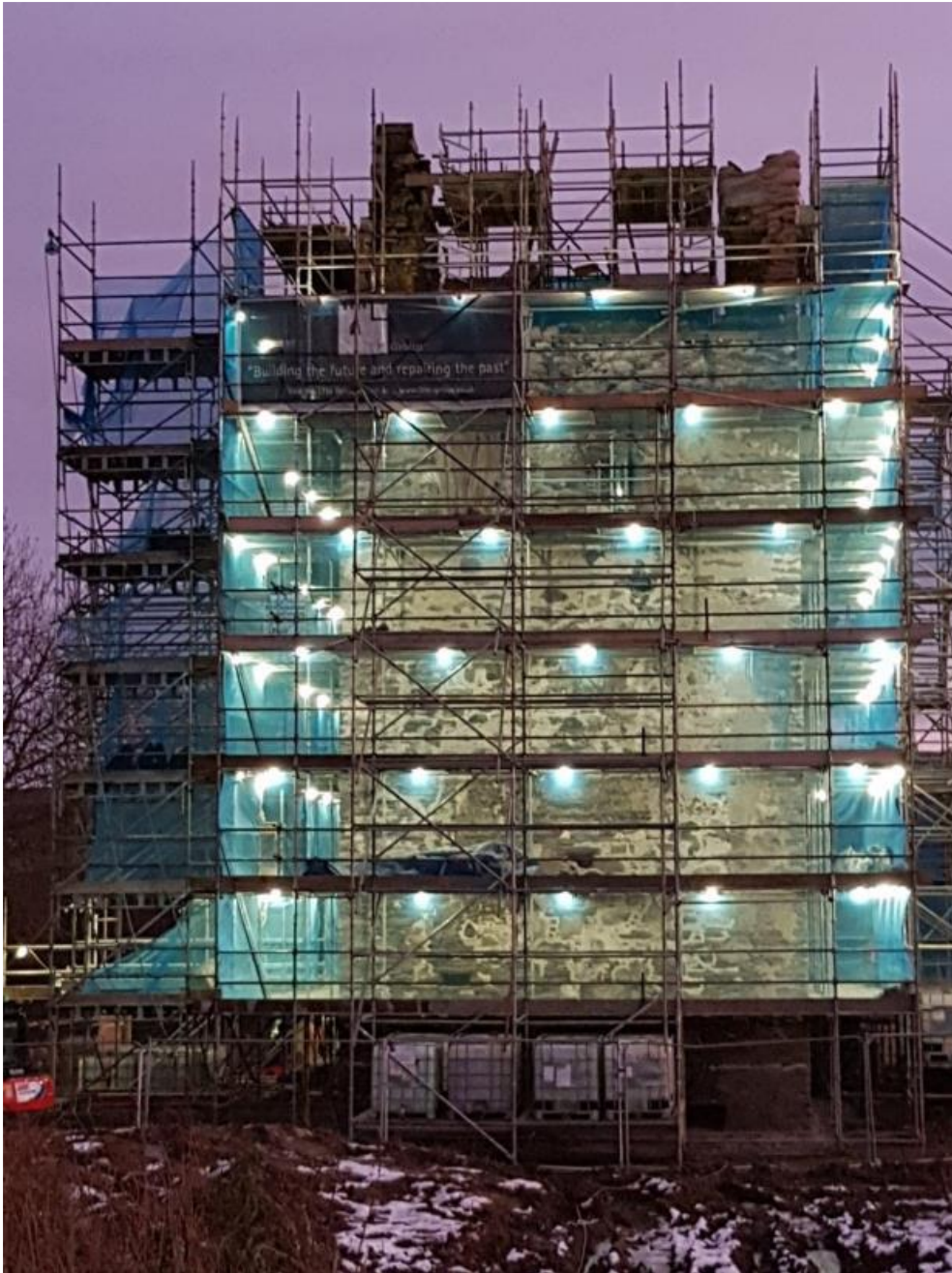
The completed scaffolding on a drear day in January 2021. The scaffold tower took more than three months to erect. It was carefully designed and placed to avoid damaging the newly discovered cobbled surface and stabilised by massive water-filled gabions.
