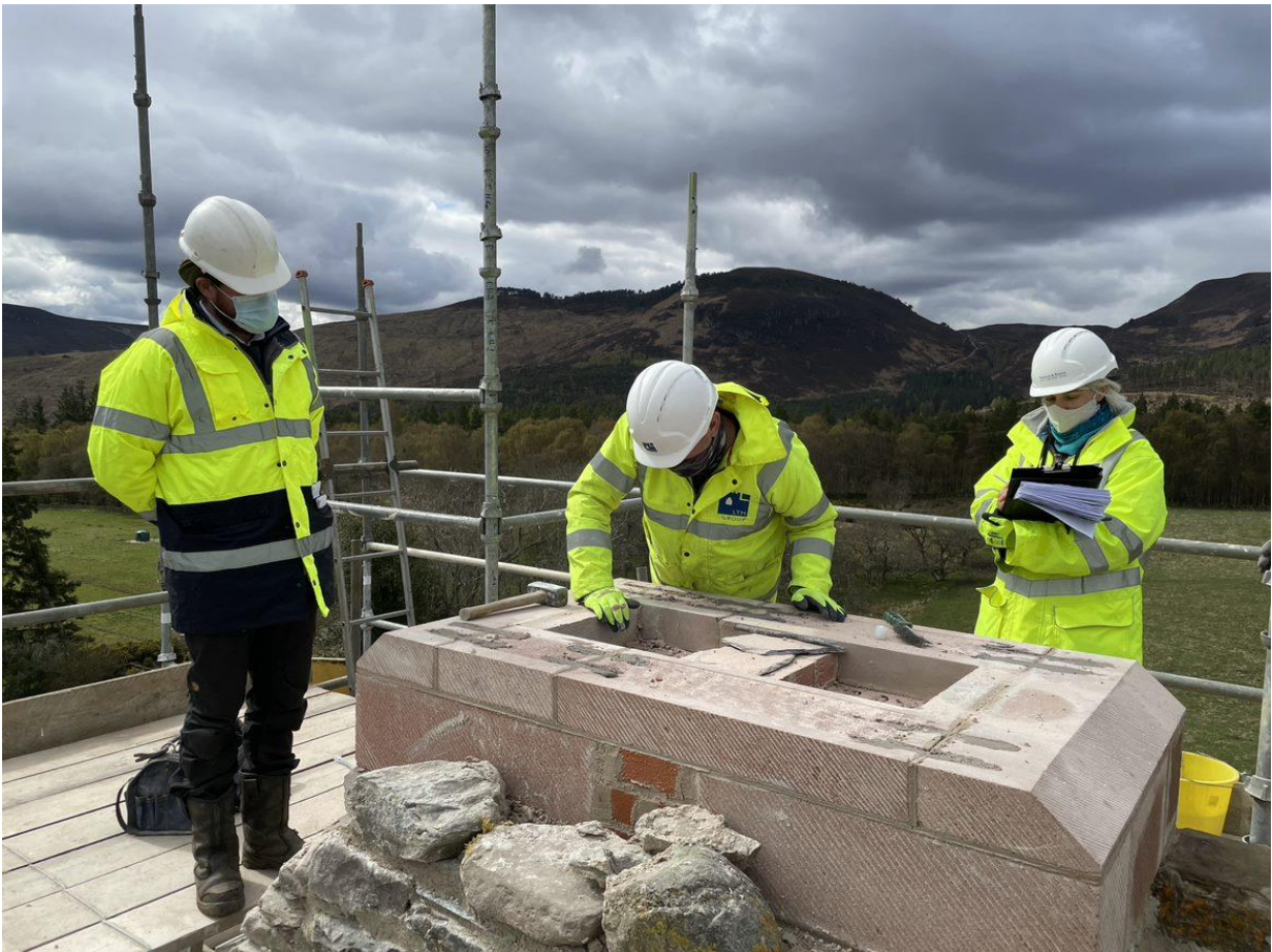
By summer 2021, masonry repairs were well underway onsite (top). Inspecting a new chimney flue carefully built around the surviving stump (below).
