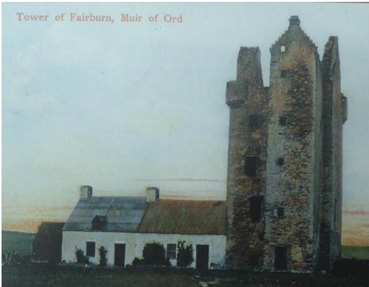
Early 20 th -century photo of Fairburn Tower, showing the dining hall in good repair and in use as two estate cottages.
