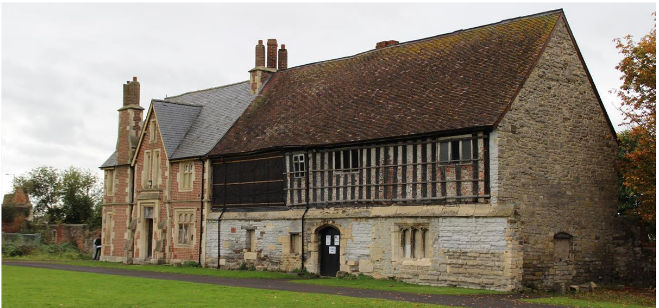
All that remains of Llanthony Secunda in Gloucester today. The buildings have also been recently restored with help from the HLF, with close contacts built between its team and Landmark's own at Llwyn Celyn.
