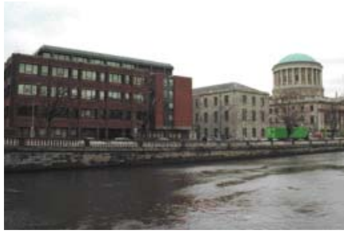
Áras Uí Dhálaigh: totally inadequate facilities
