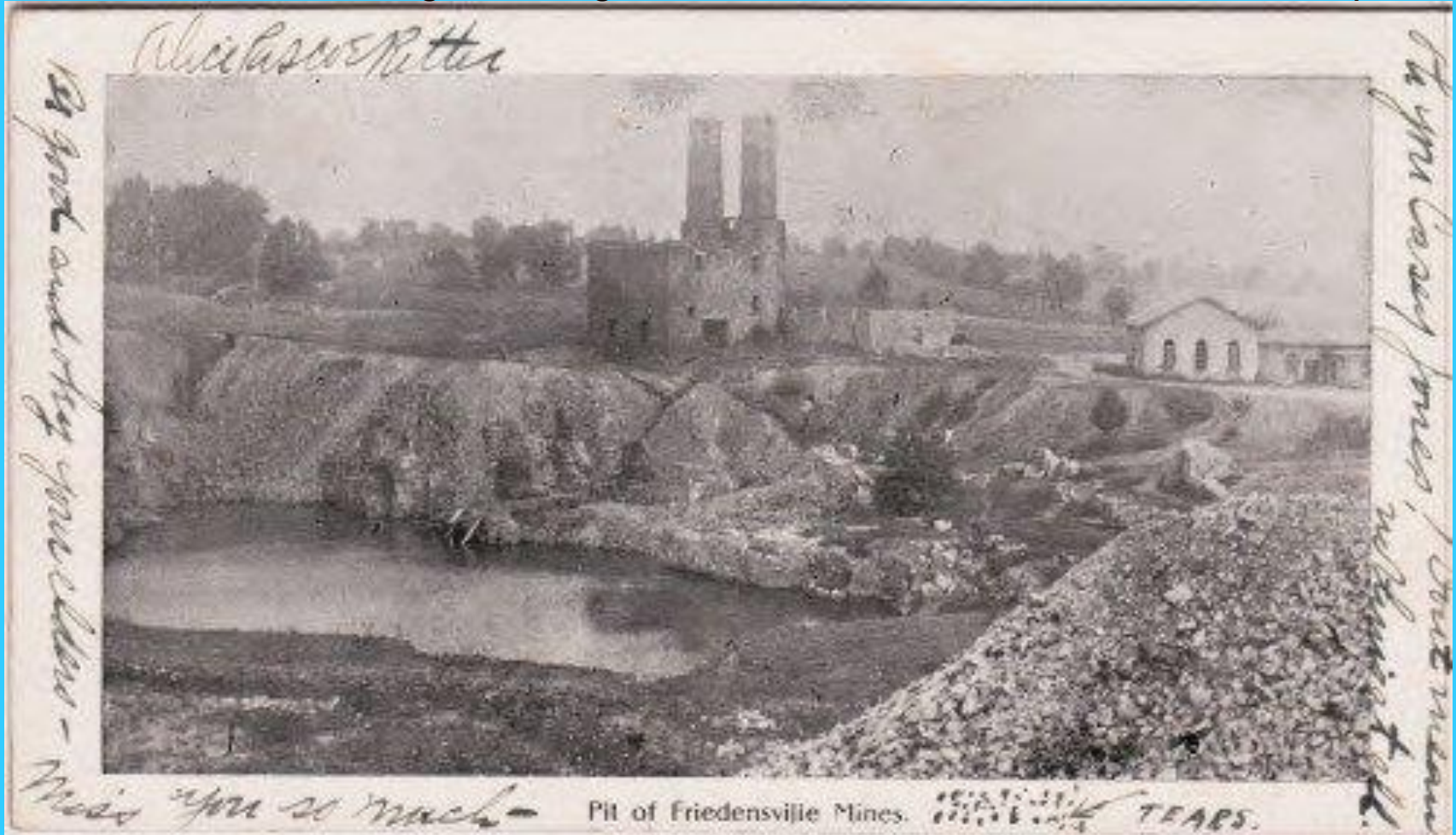
(Left to right) Engine House, Boiler House, and Mine Office
