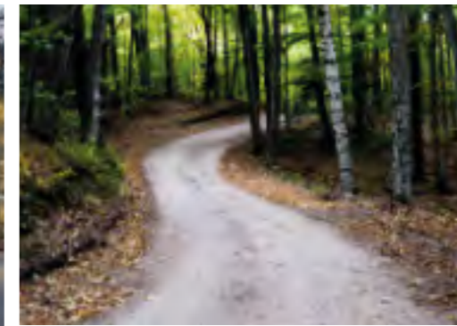
Gravel bound access road
