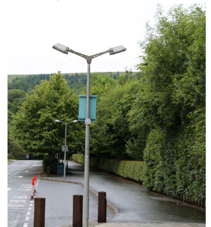
Double headed lighting columns used in Loch Lomond Shores ●
