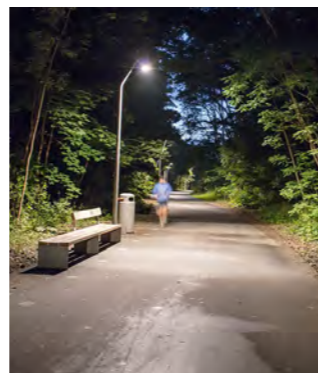
Light posts along key routes
