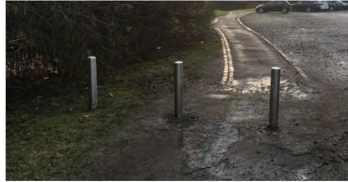
Brushed steel bollards to pedestrian routes ●
