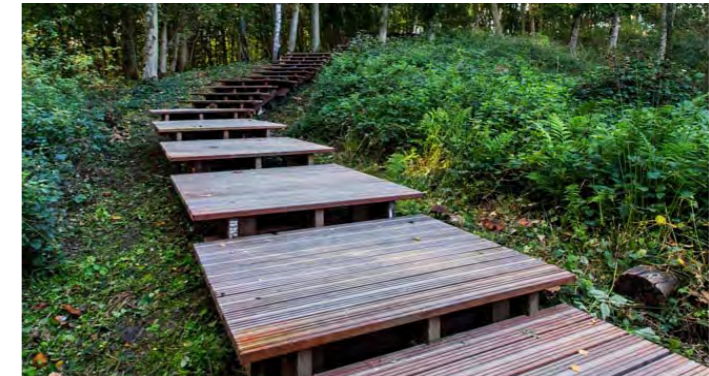
Timber board-walks elevated off ground level
