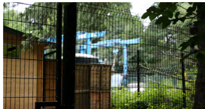
High steel mesh, security fence ●
