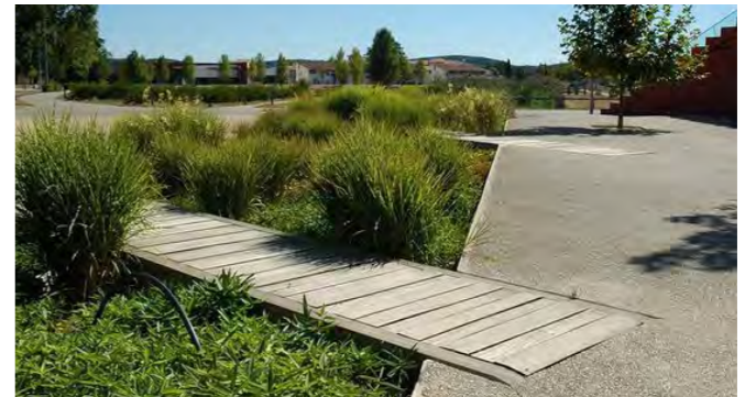
SUD's planted strips within hard landscape areas
