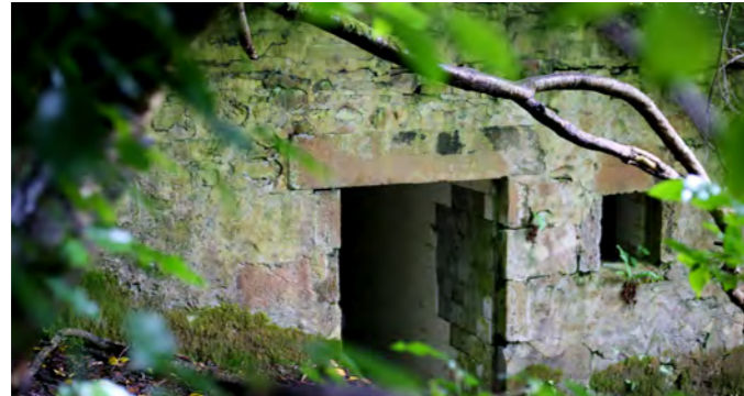
Restoration of derelict buildings
