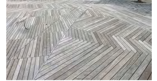
Areas of timber decking
