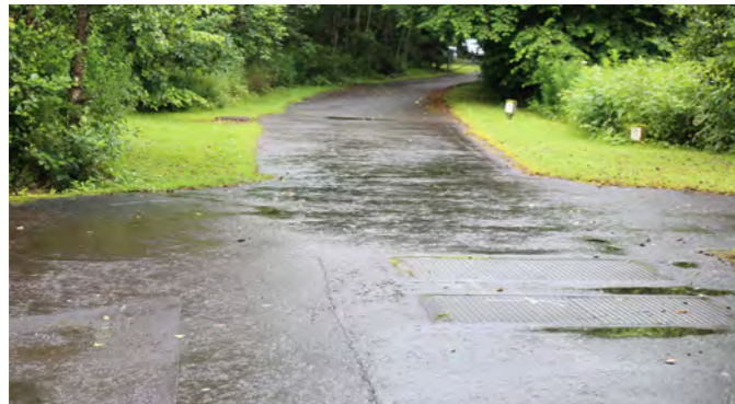
Asphalt along key access routes
