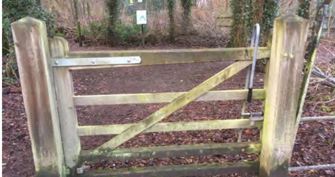
Rustic timber post and rail gateway ●
