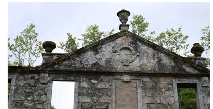
09 - Woodbank historical facade
