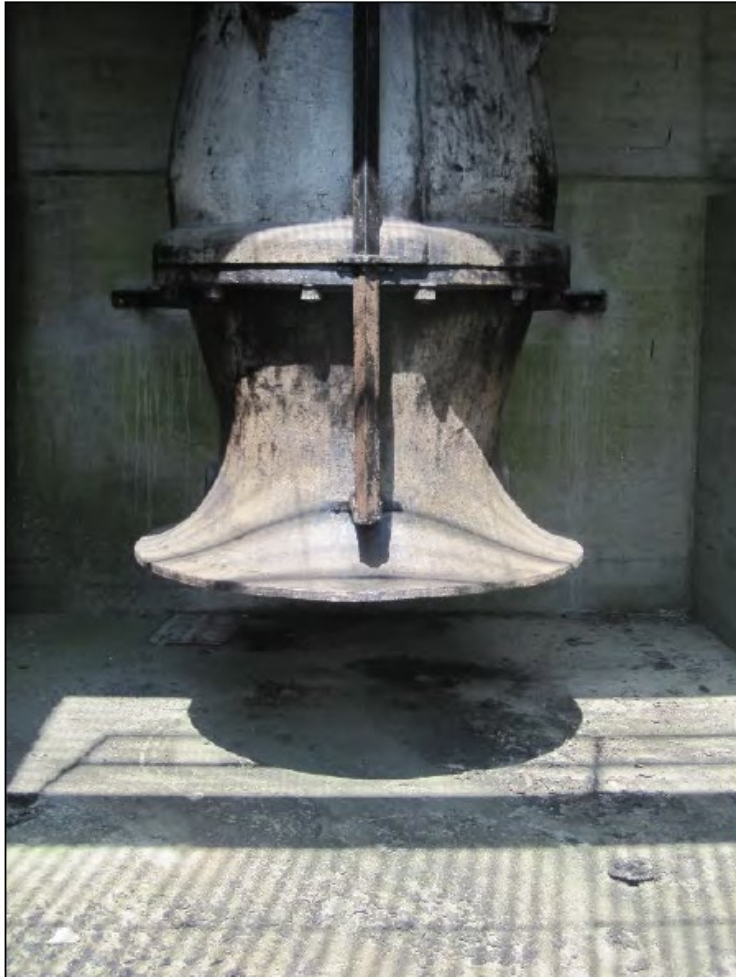
(Courtesy of USACE Louisville District)
