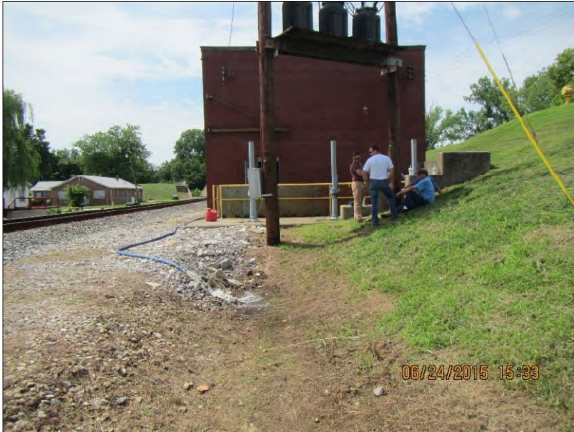
(Courtesy of USACE Louisville District) Figure 9-2. Pump station at landside toe.
