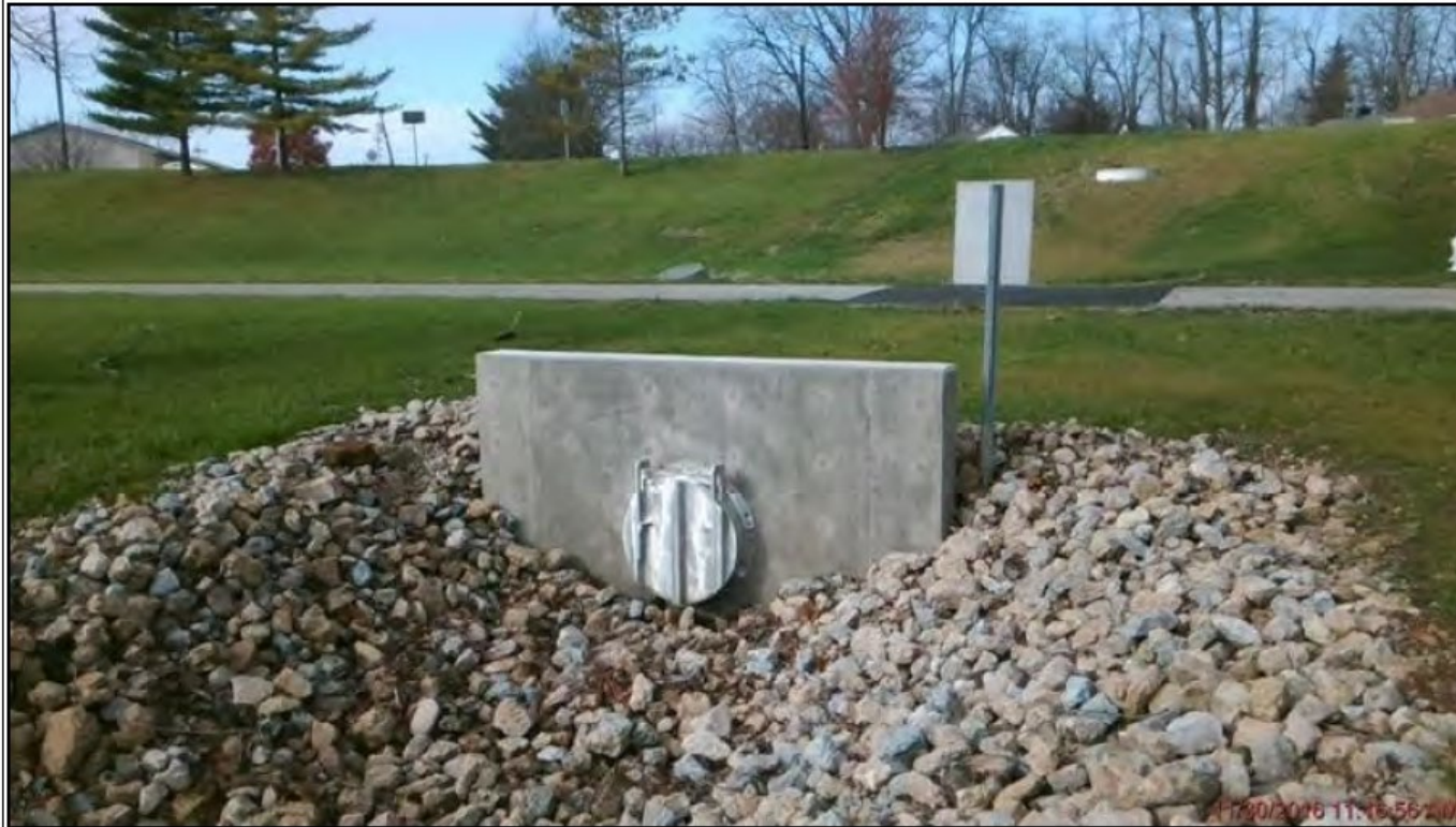
(Courtesy of USACE Louisville District)
