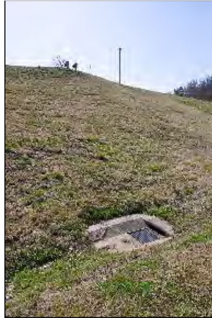
(Courtesy of USACE Louisville District)
