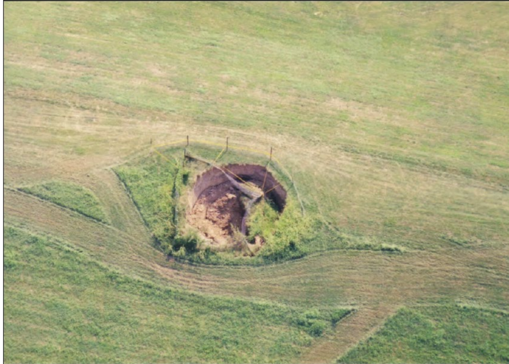
(Courtesy of USACE Louisville District)
