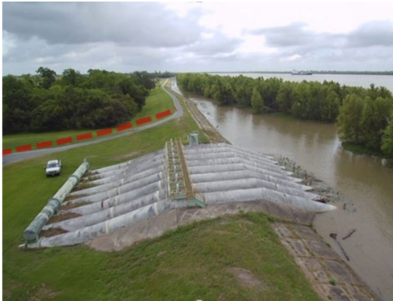
Figure 5-8. Elevated non-passable pipes prevent vehicular crossing.
