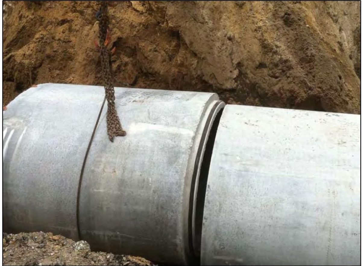
(Courtesy of American Concrete Pipe Association) Figure 3-1. Installation of precast RCP.
