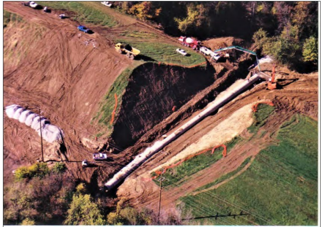
(Courtesy of USACE Louisville District)
