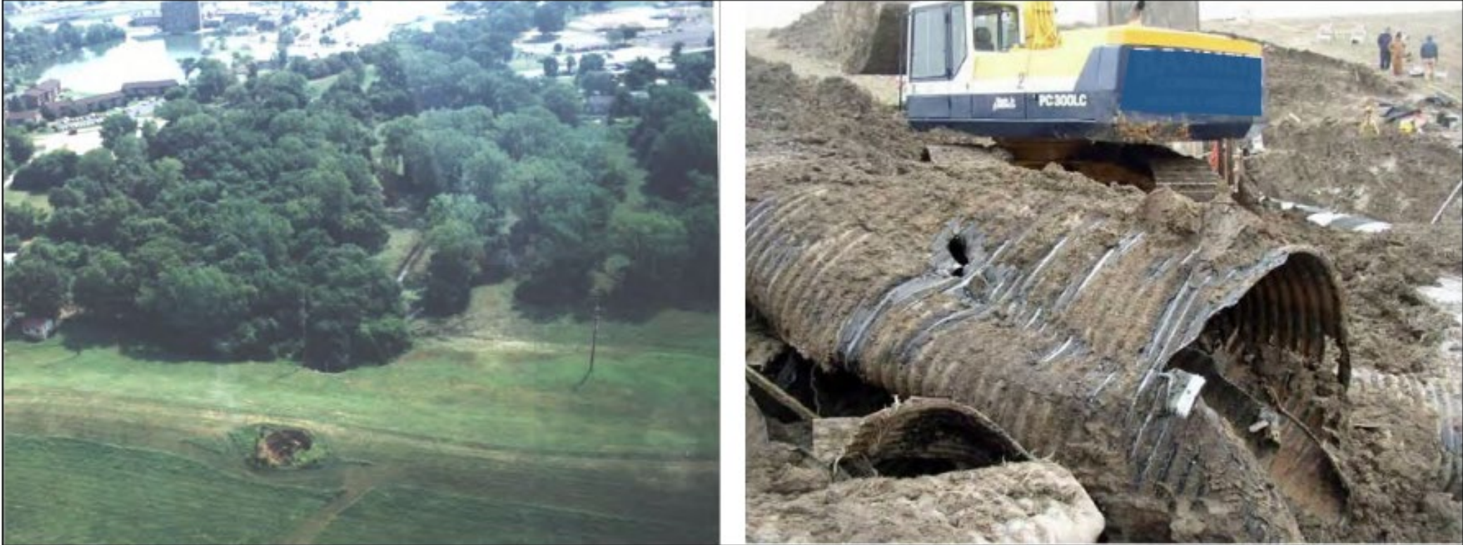
(Courtesy of USACE Louisville District)
