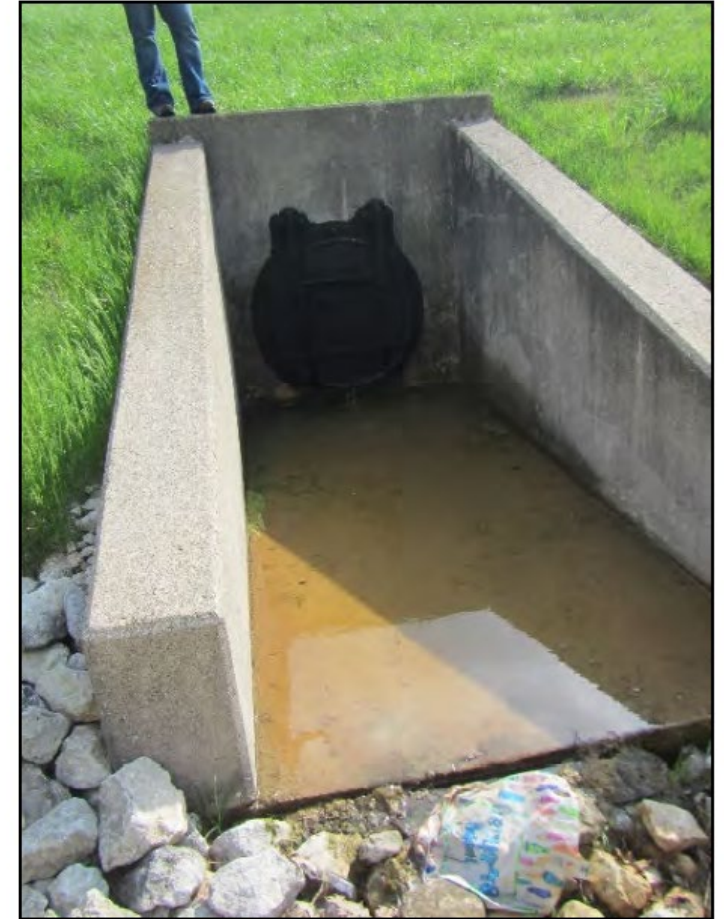
(Courtesy of USACE Louisville District)
