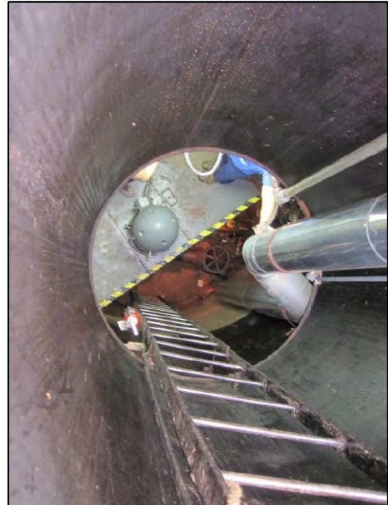
(Courtesy of USACE Louisville District)
