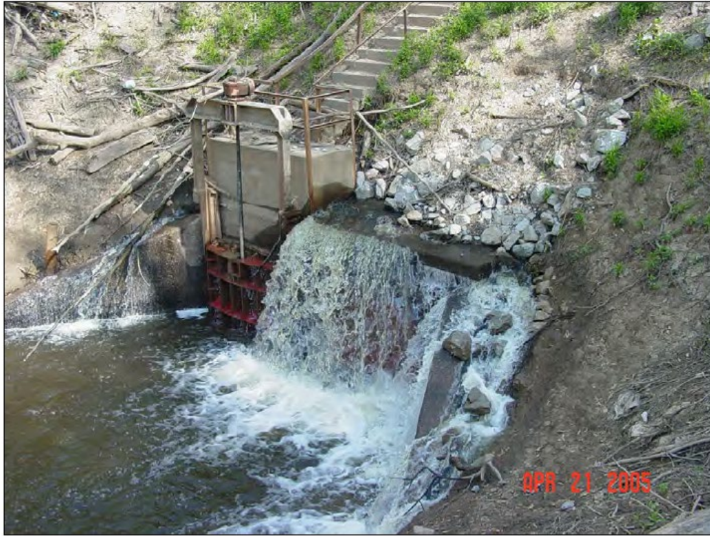
(Courtesy of USACE Louisville District)
