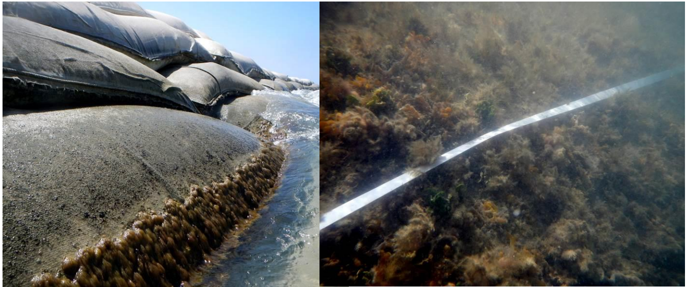
Figure 4. The intertidal zone on the sand bag groin is coated in macroalgae (left photo) that extends as macroalgal and cyanobacterial growth along the base of the west side of the groin (right photo).
