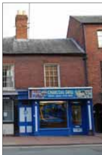
No 8A Teme Street
