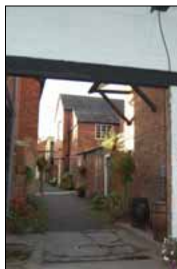
Arch at No 31 Teme Street
