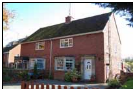
No 9-10 Pembroke Avenue
