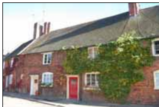
No 13-14 Church Street
