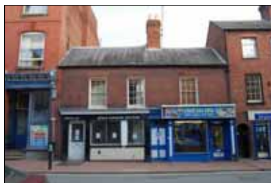
Varying roofscape along Teme Street
