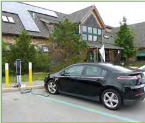
The electric charging station at Joppa Flats Education Center in Newburyport is powered by the center's rooftop solar panels.
