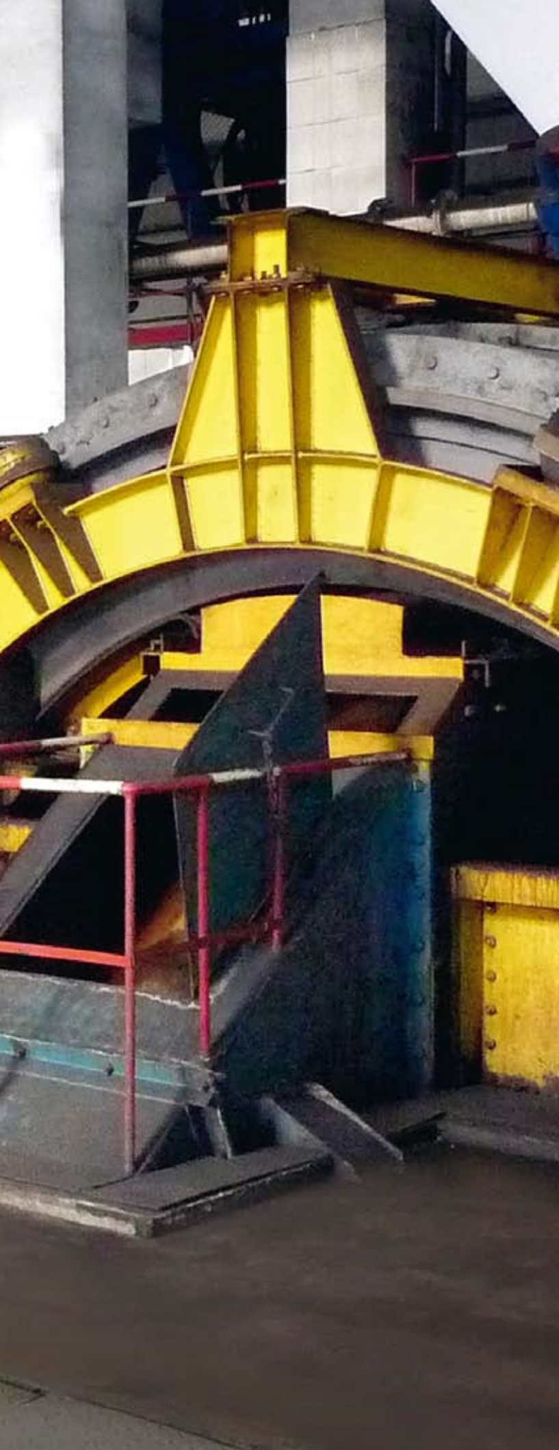
ROMJIG plant for run of mine coal, China
