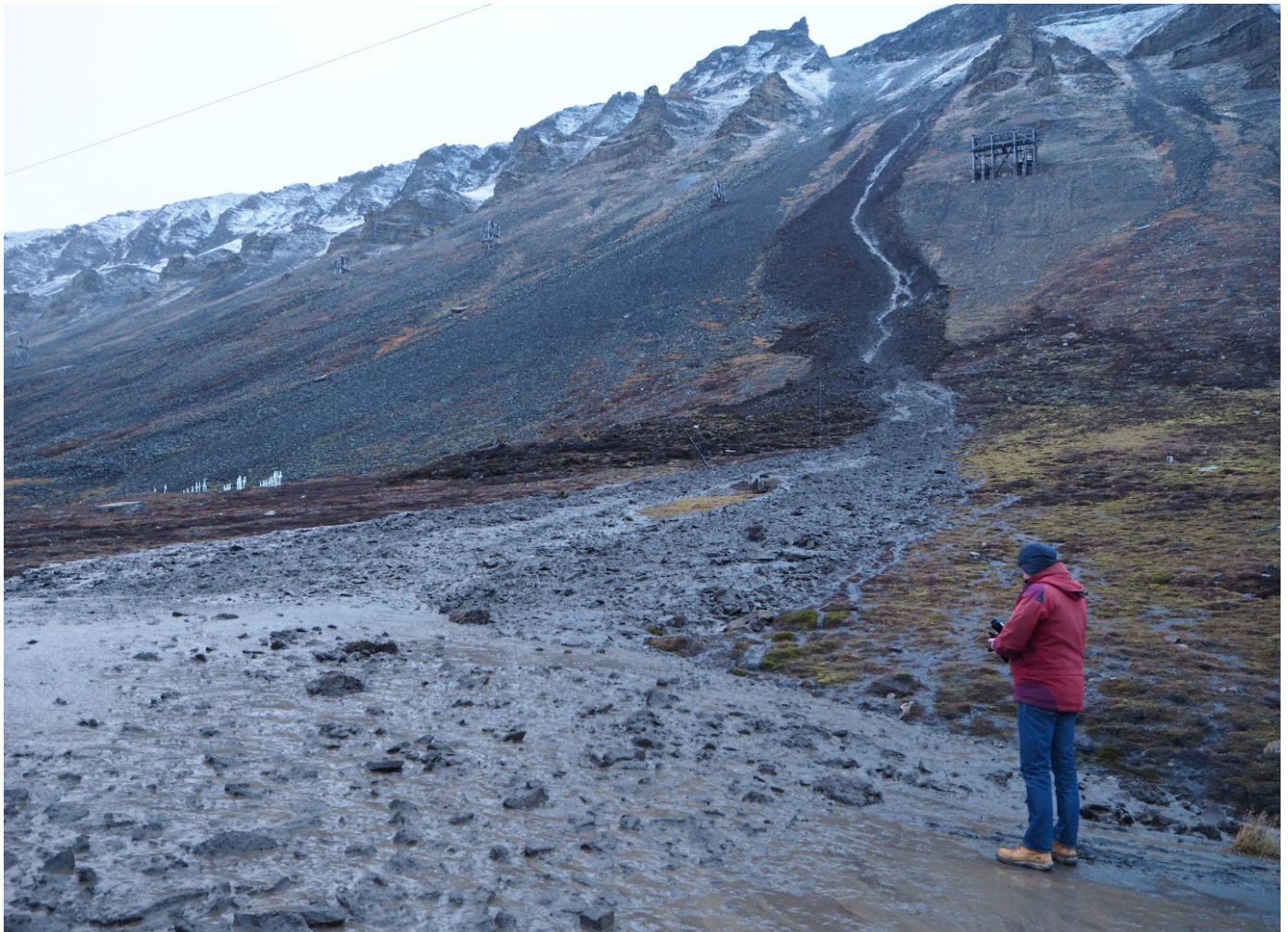
Figure 10.3.3 Slope failures at the Longyearbyen cemetery 16 October 2016 causing a slump and associated debris flow crossing the road. Photo: Hanne H. Christiansen.
