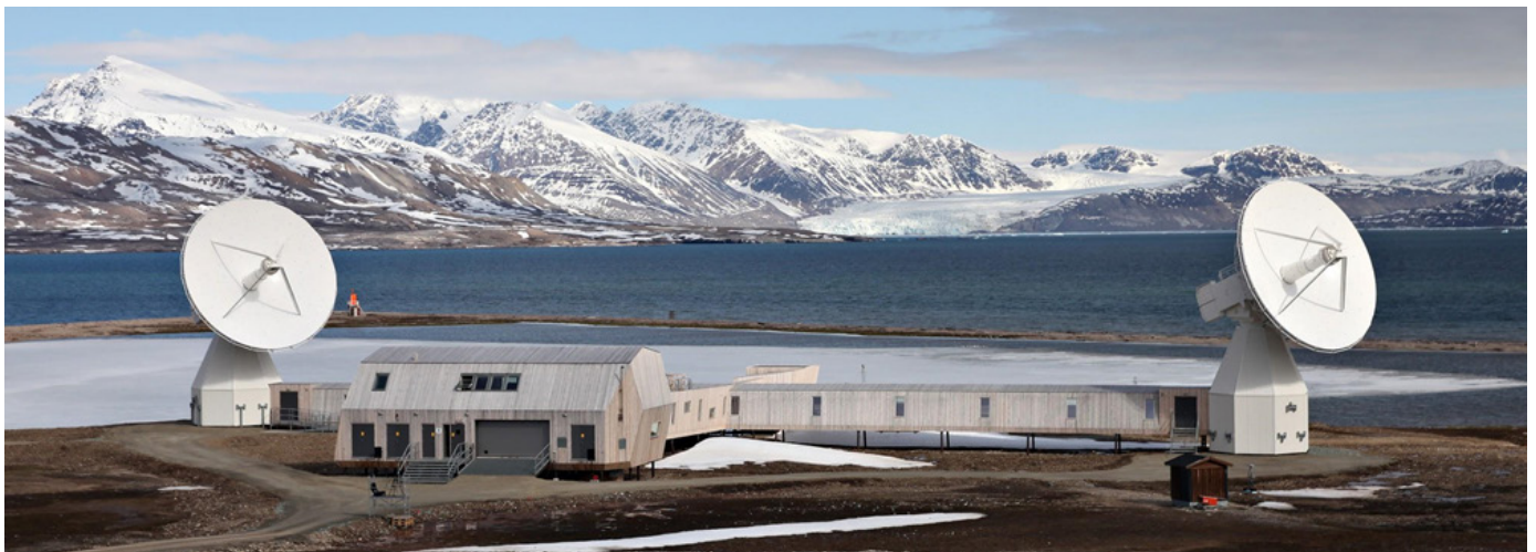
Figure 3.6.2 The Earth observatory at Ny-Ålesund which is a core geodetic site, i.e. a number of different geodetic instruments are collocated. The site is part of a global network that is of fundamental importance for determining accurate measurements of sea level from satellite altimetry. The twin VLBI telescope is pictured. Photo: Bjørn-Owe Holmberg
