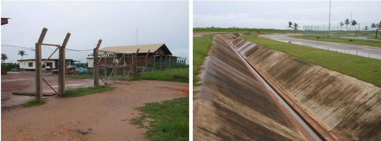
Figure 4.4 VRA's Scrap Yard & Storm Drain
