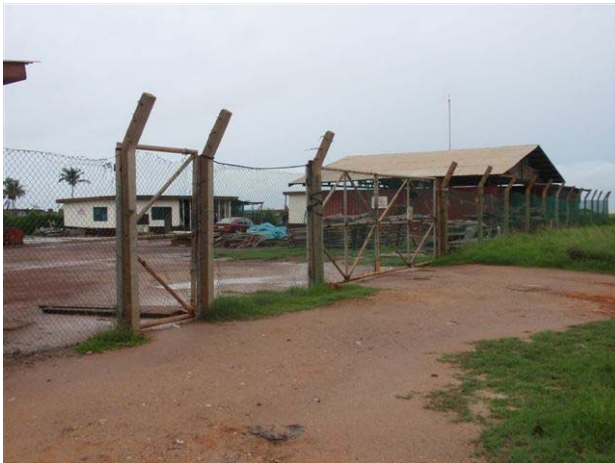
Figure 4.4 VRA's Scrap Yard & Storm Drain
