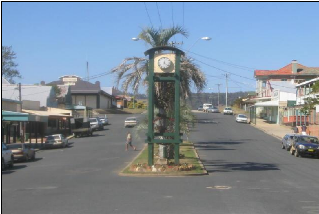
Figure 8.6: High Street, Bowraville (Bowraville Conservation Area)
