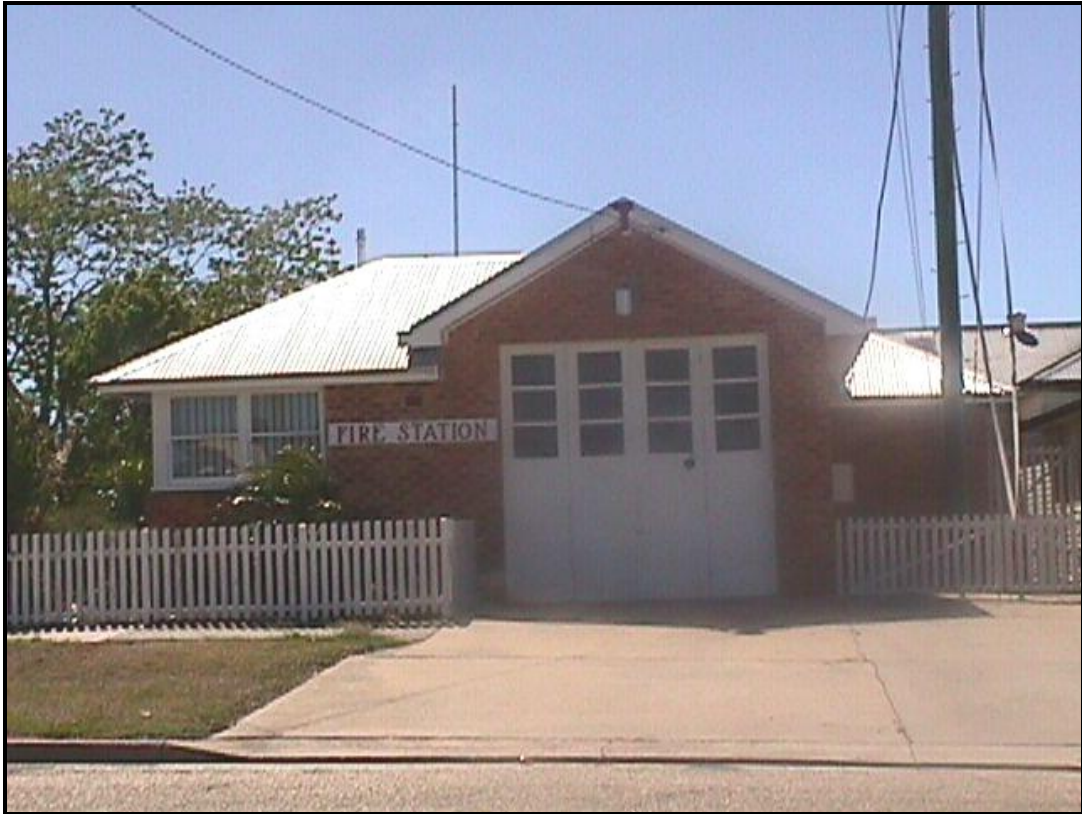
Figure 8.7: Fire Station, 55 High Street, Bowraville
