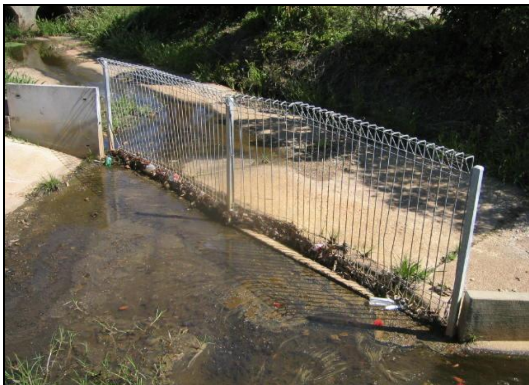
Figure 3.7: Pollutant Trap on Beer Creek, Nambucca Heads
