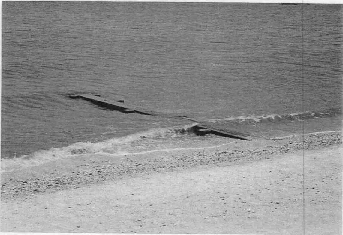
2. TIMBER BULKHEAD GROIN LOCATED AT WASHINGTON AVENUE
