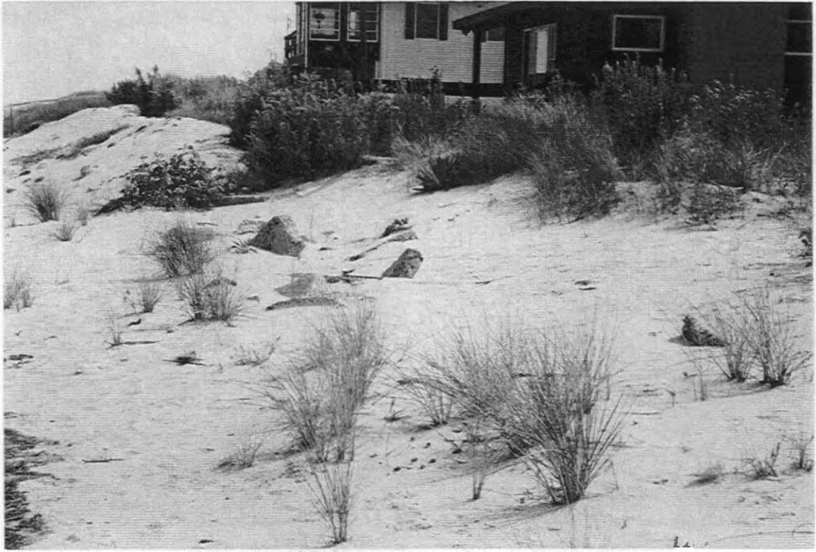
7. CONCRETE RUBBLE REVETMENT LOCATED NORTH OF ALABAMA AVENUE
