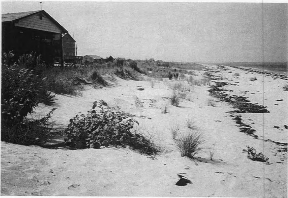
6. CONCRETE RUBBLE REVETMENT LOCATED NORTH OF ALABAMA AVENUE
