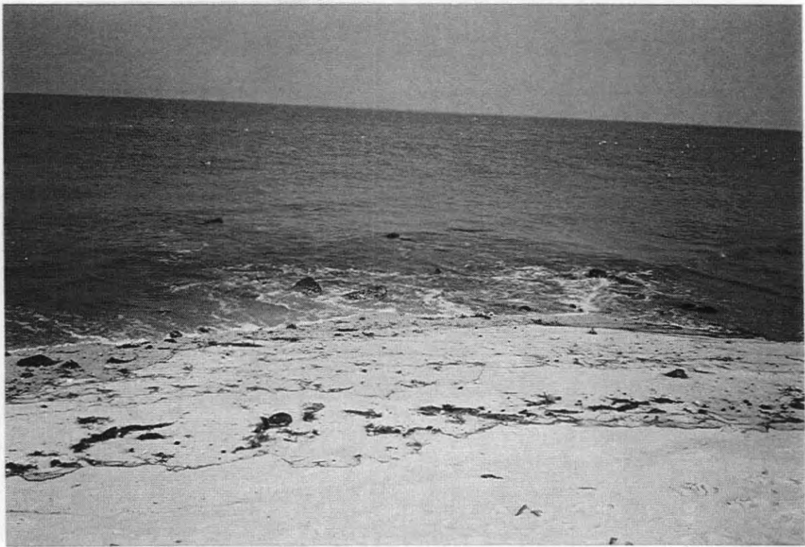
4. CONCRETE RUBBLE GROIN LOCATED AT GEORGIA AVENUE
