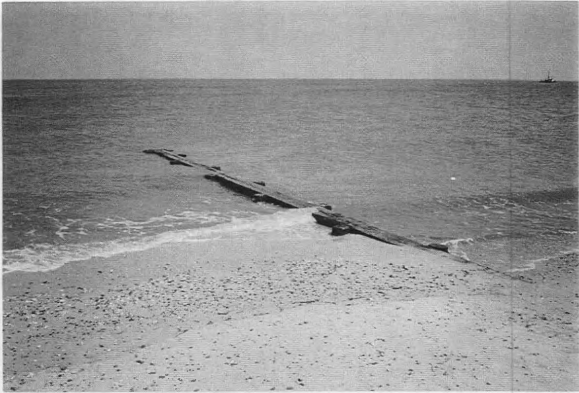
1. TIMBER BULKHEAD GROIN LOCATED AT ADAMS AVENUE
