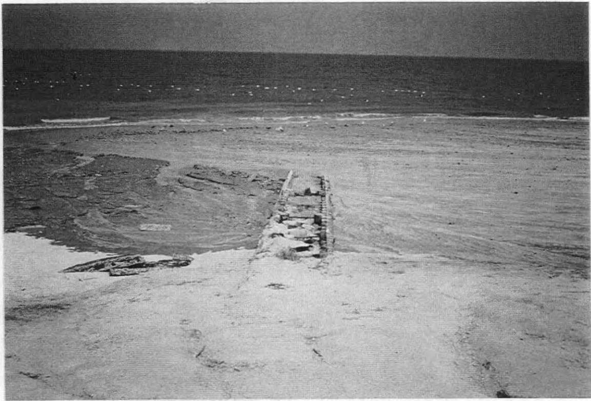
3. STONE FILLED TIMBER CRIB GROIN LOCATED AT NORTH CAROLINA AVENUE
