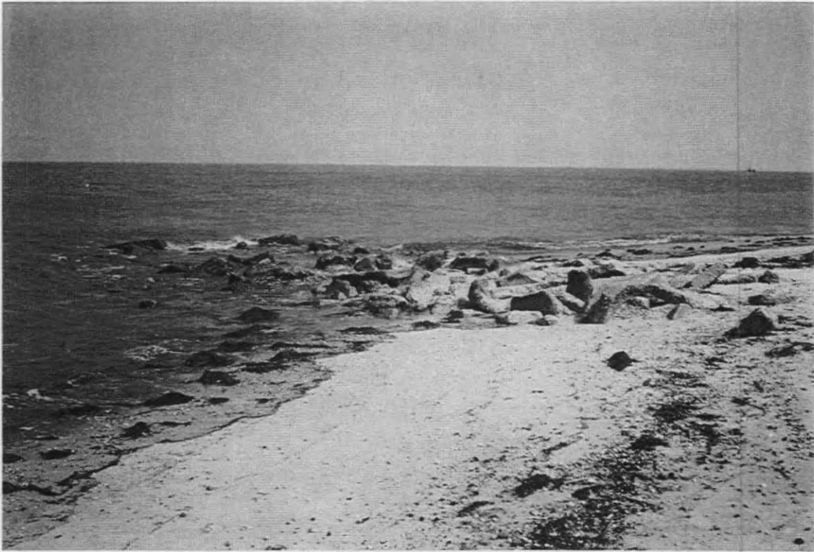
5. CONCRETE RUBBLE GROIN LOCATED AT ALABAMA AVENUE
