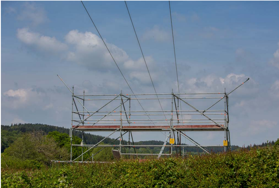
Photograph showing typical temporary scaffold tower
