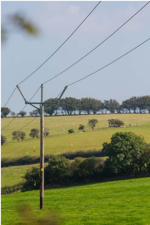
Photograph showing typical completed pole location
