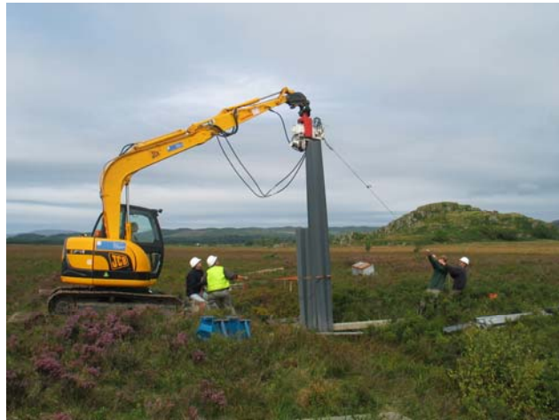
Excavator driving in dams
