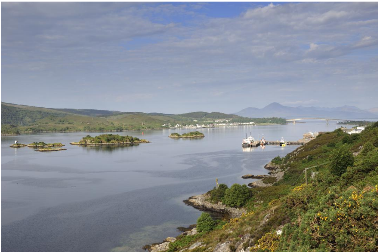
Kyleakin and the Skye bridge from Kyle of Lochalsh, Isle of Skye. ©Lorne Gill/NatureScot
