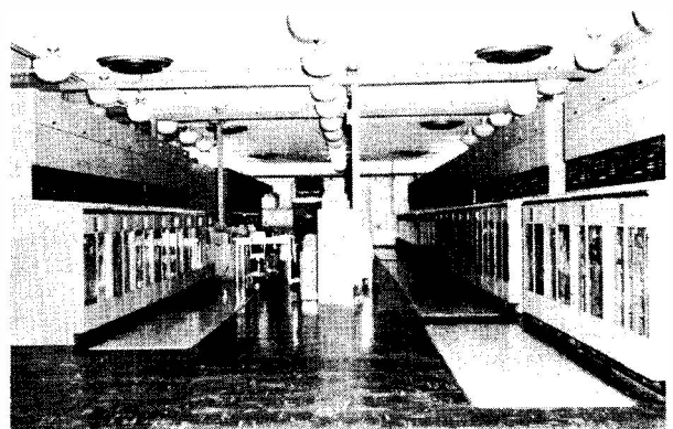
31.31 Figure 10-40.— Automatic relay center.
