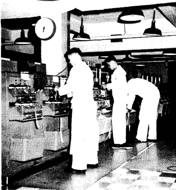
31.30 Figure 10-39.—Receiving and transmitting consoles at a torn-tape relay center.
