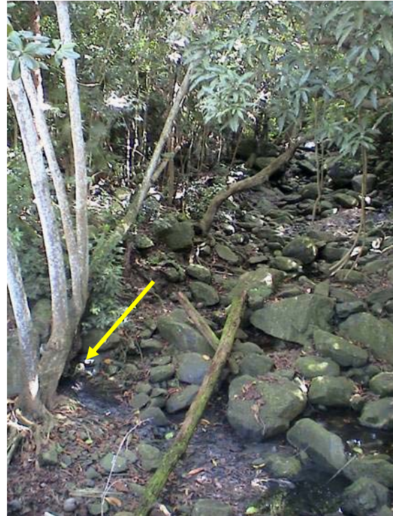
Figure 8. Sewage input in Dorothea gut (yellow arrow)
