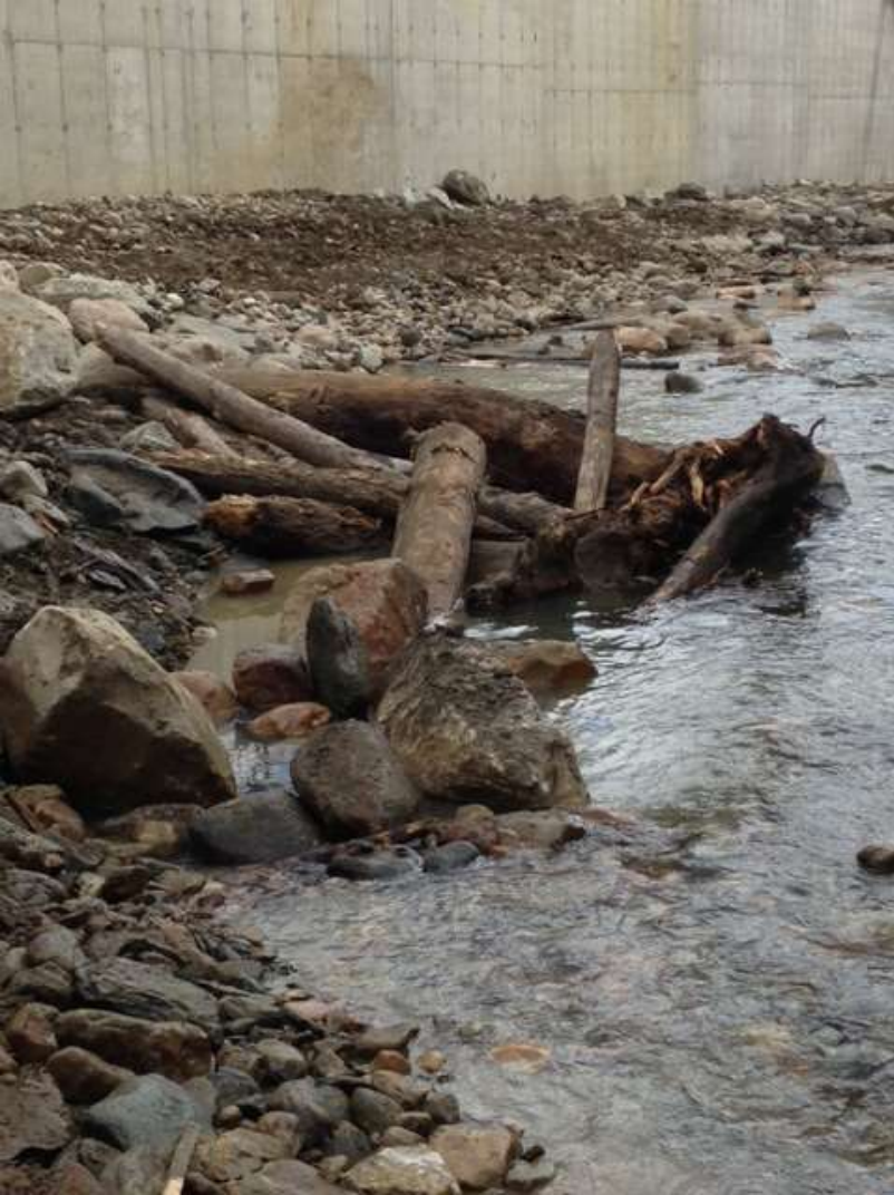
Large Wood Deflector at Retaining Wall Repair Route 9, Westfield Brook - Cummington, MA MMI, 2017
