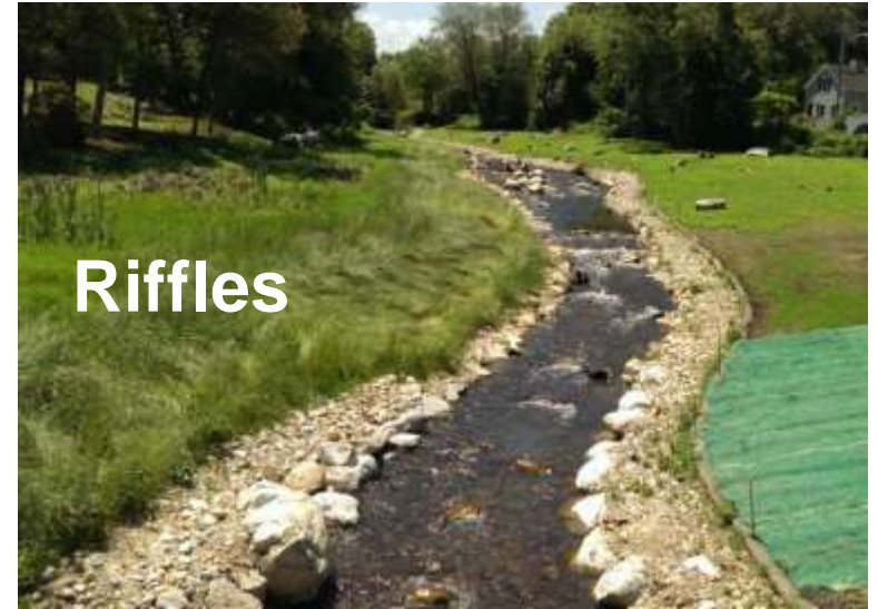
Plymco Dam Channel Restoration (J. MacBroom, 2015)
