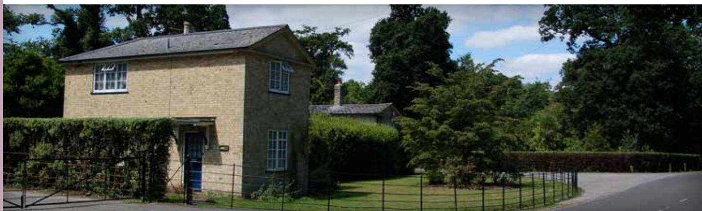
Traditional estate railings around the Exbury Estate lodges
