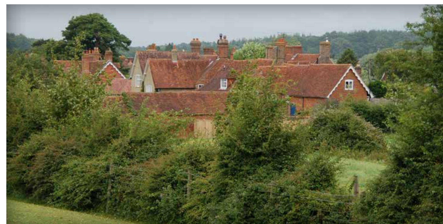
The rhythm of clay roof tiles, chimneys and steeply pitched roofs in Beaulieu
