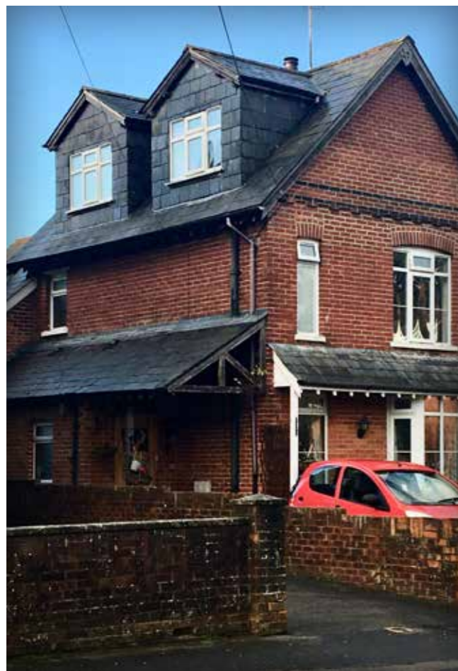
The large dormers feature wide cheeks, and appear heavy and out of proportion with the scale of the cottage
