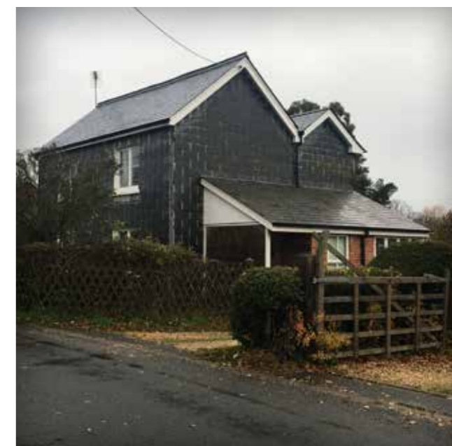
Side and rear extension subservient to the original cottage
