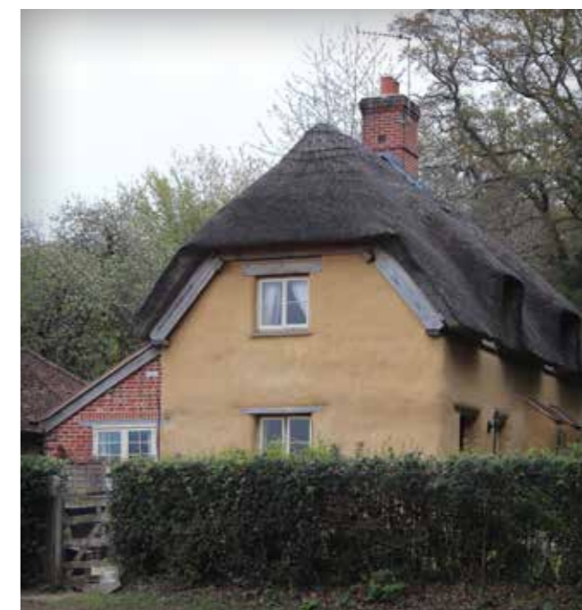
A cottage in Woodgreen rebuilt in cob after fire damage
