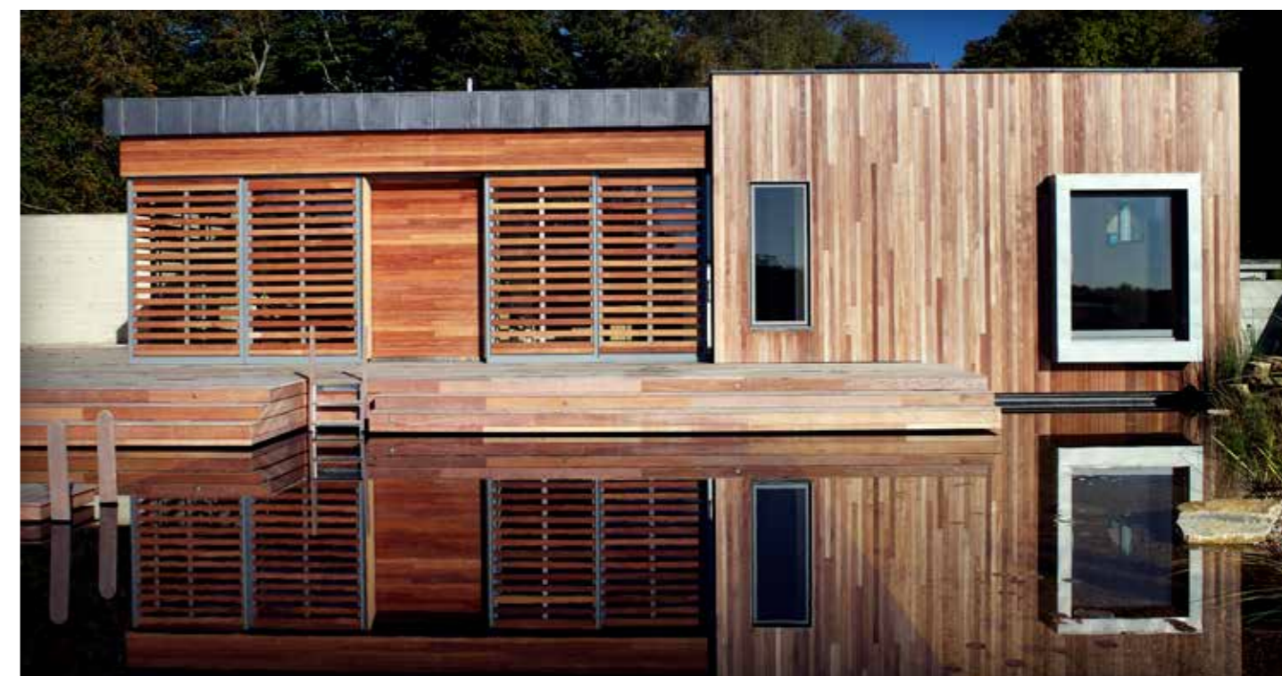
Effective use of louvres on this contemporary design to provide shading and reduce the impact of light spill from the large windows
