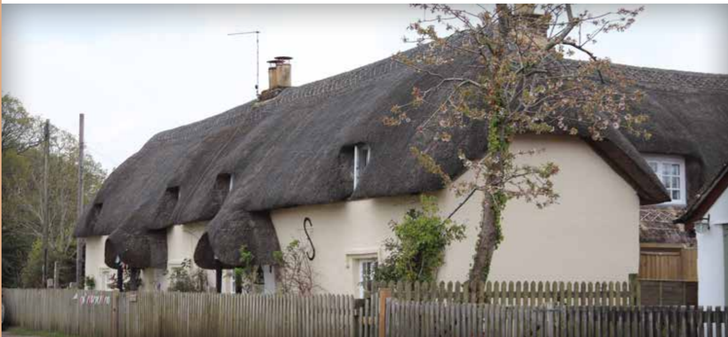
A pair of lime plastered cob cottages under a thatched roof with a traditional simple flush ridge,, Hale
