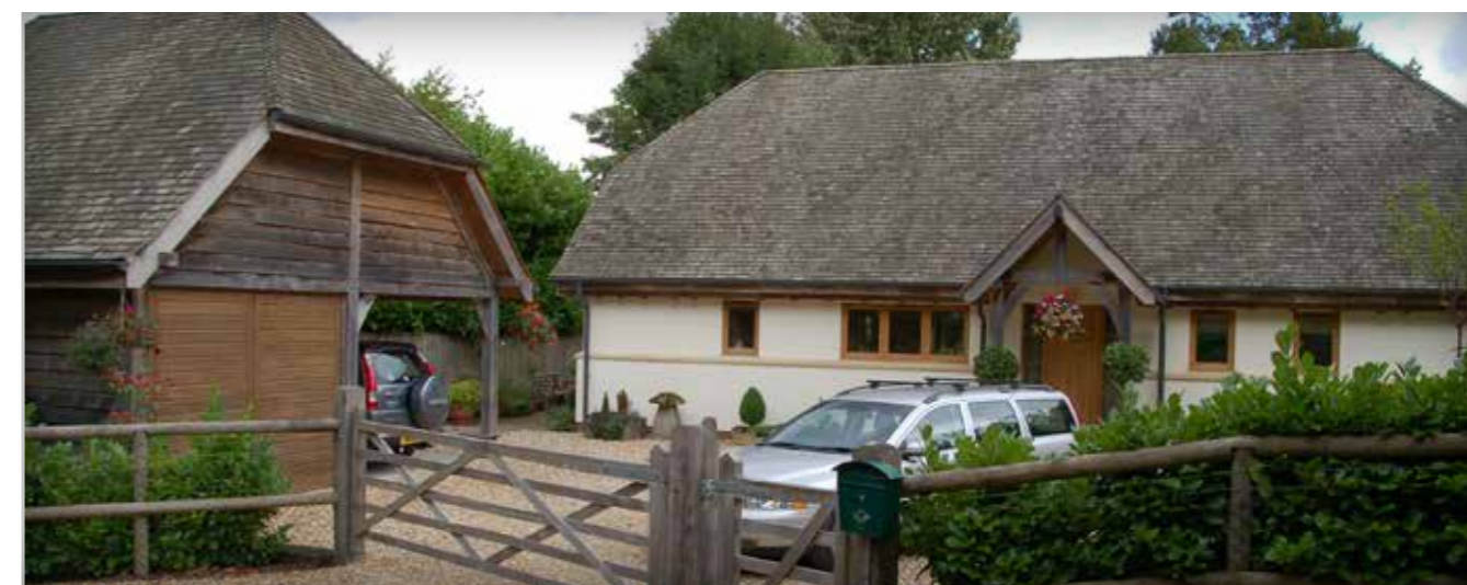
A shingle roof on a new build cottage, Burley
