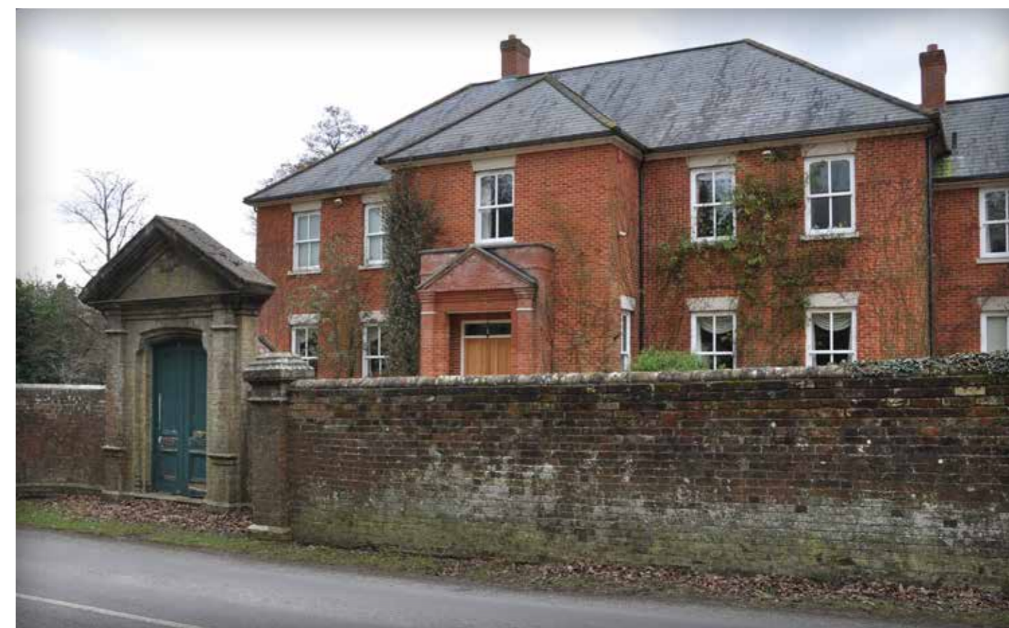
An example of a locally listed small country house built in a formal architectural style, with a grandiose pedimented gateway
