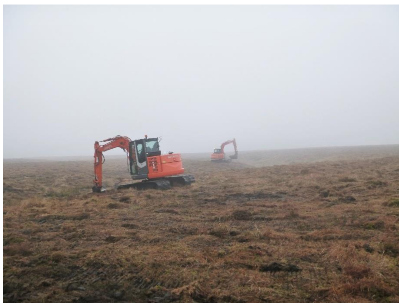
Figure 3 The contractor on site and delivering peatland restoration.
