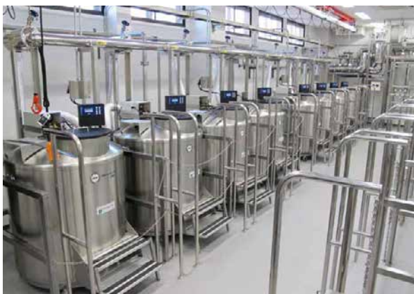
Figure 2. Cryogenic storage system. Liquid nitrogen tanks are monitored 24 hours a day and are refilled automatically.
