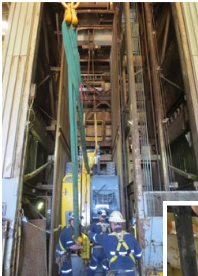
Mining rope install
