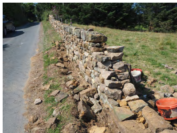
Fig.19 Dry stone wall under repair, Raw
