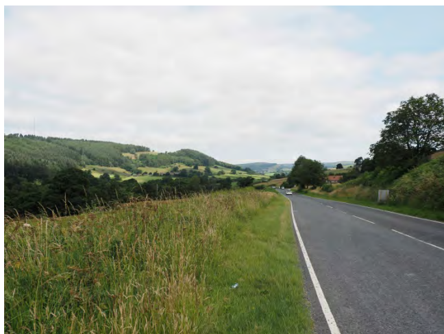
Fig.49 A typical scene in LCA 2b, looking North along Bilsdale from the B1257
