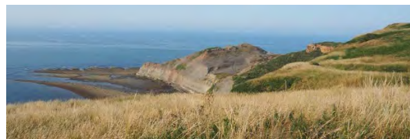
Fig.138 Historic alum mining and processing has totally changed the shape of the headland at Kettleness
