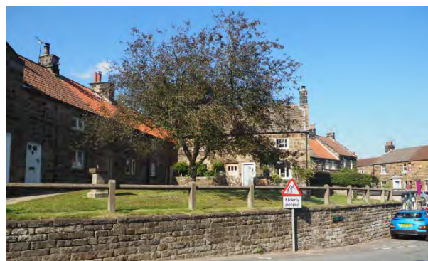
Fig.117 Vernacular buildings in Castleton village
