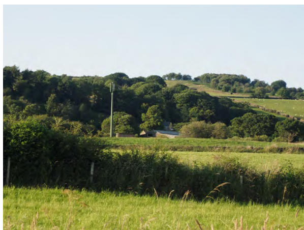
Fig.22 Well-sited and designed mobile phone mast, Houslyke
