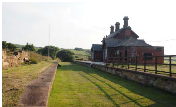
Fig.76 Former station and platforms at Kettleless
