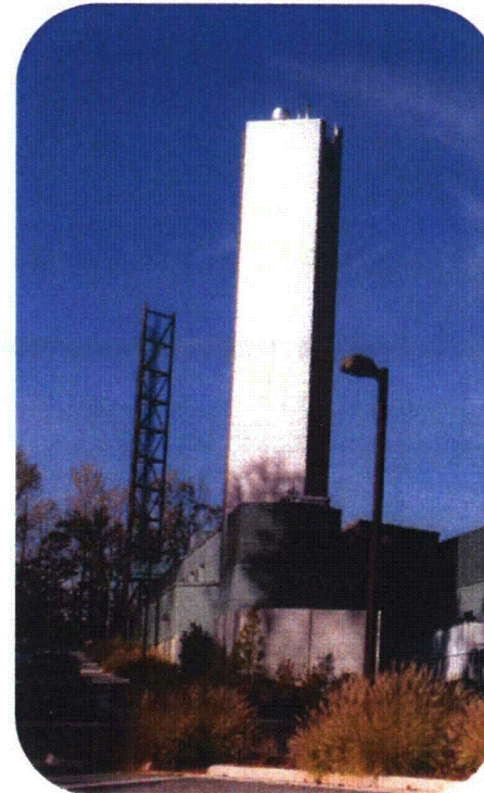
Full height Integrated Systems Test Facility Bedford, Virginia
