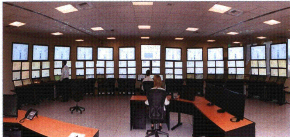
NuScale Control Room Simulator
