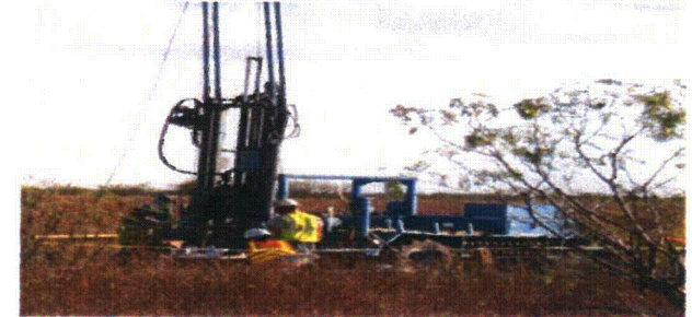
Bore hole drilling at Clinch River
