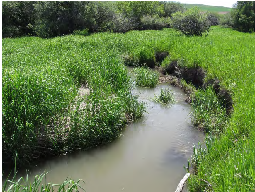
FIGURE 7. NON-NATIVE PLANTS WITH SHALLOW ROOT SYSTEMS CAN LEAD TO BANK FAILURE.
