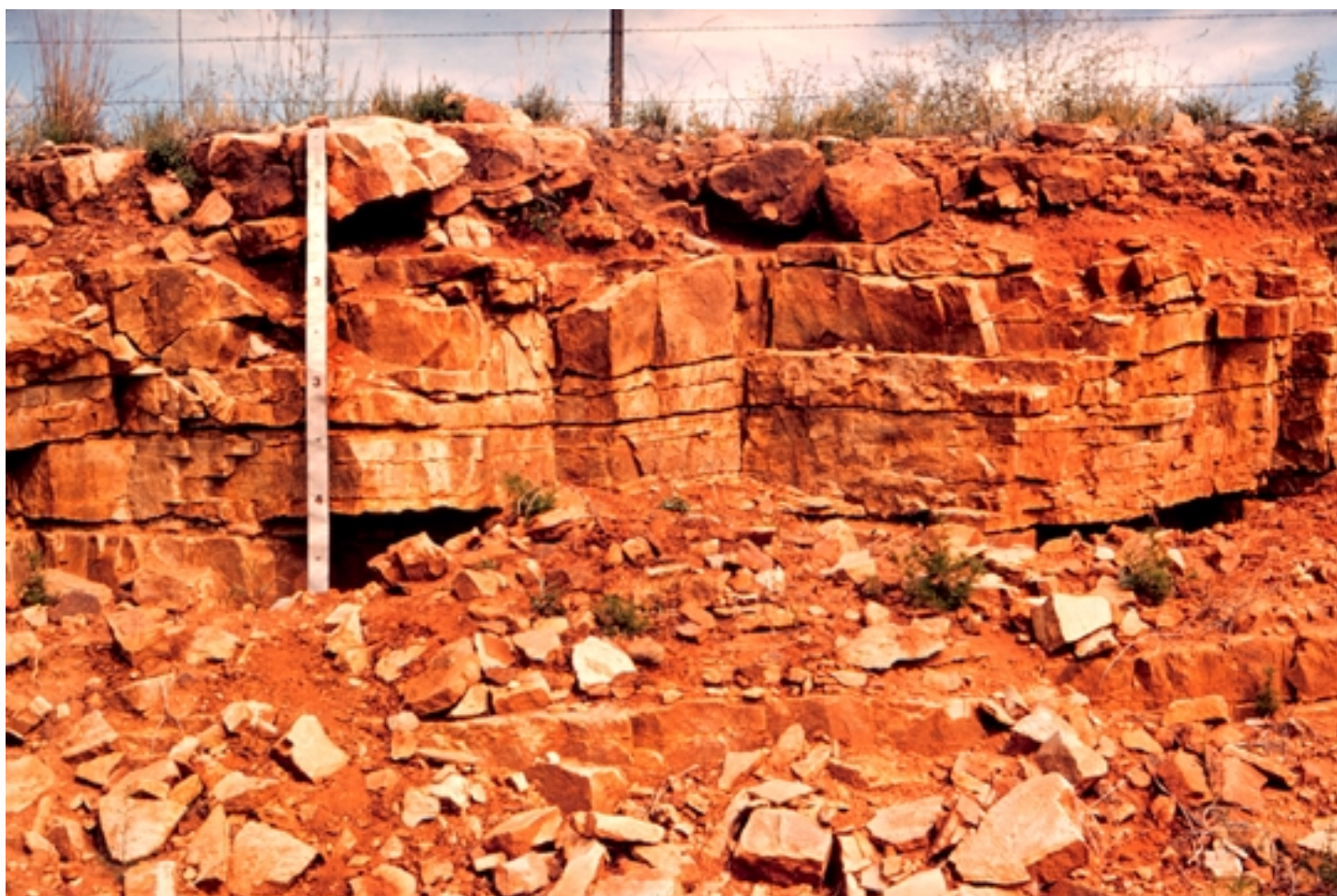
Photo 39.—Fractured lithic contact. Vertical fractures are greater than 10 cm. Sandstone is below the lithic contact.
