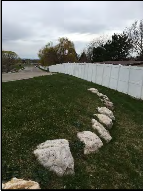
Photo 3: Another portion of Site 1 of the proposed project. The pipeline, which would be replaced as part of the project, is buried from the pump station and runs south along the edge of the right-of-way toward the existing stormwater detention basin.
