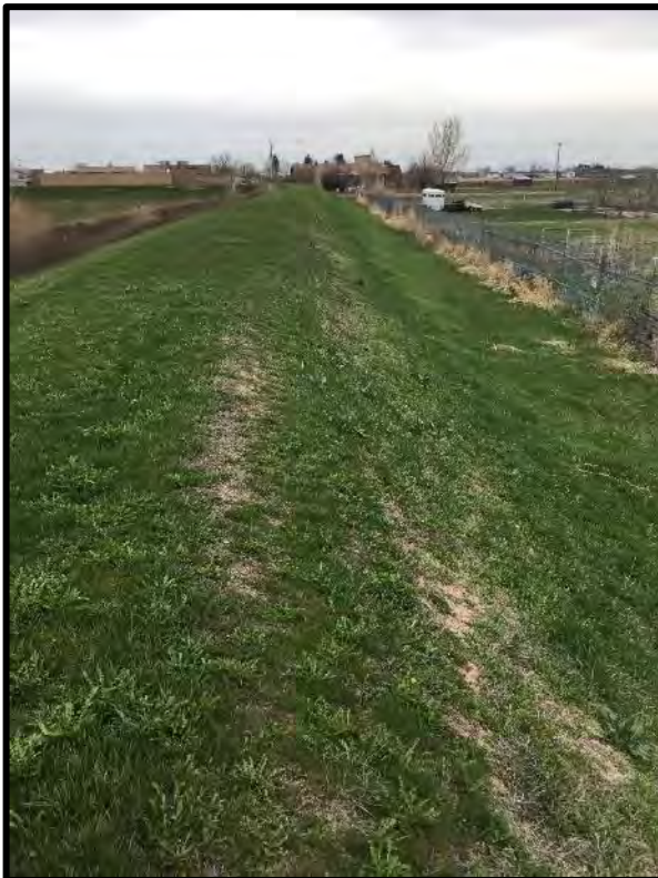
Photo 6: From the northwest corner of the existing stormwater basin, the proposed irrigation pipeline would turn south and continue along the outside edge of the detention basin berm (Site 2).
