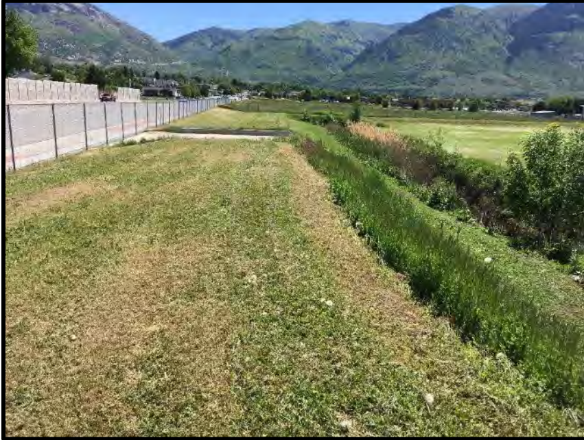
Photo 5: From the northeast corner of the existing stormwater detention basin, the proposed irrigation pipeline would be placed around the outside edge of the detention basin berm (Site 2).
