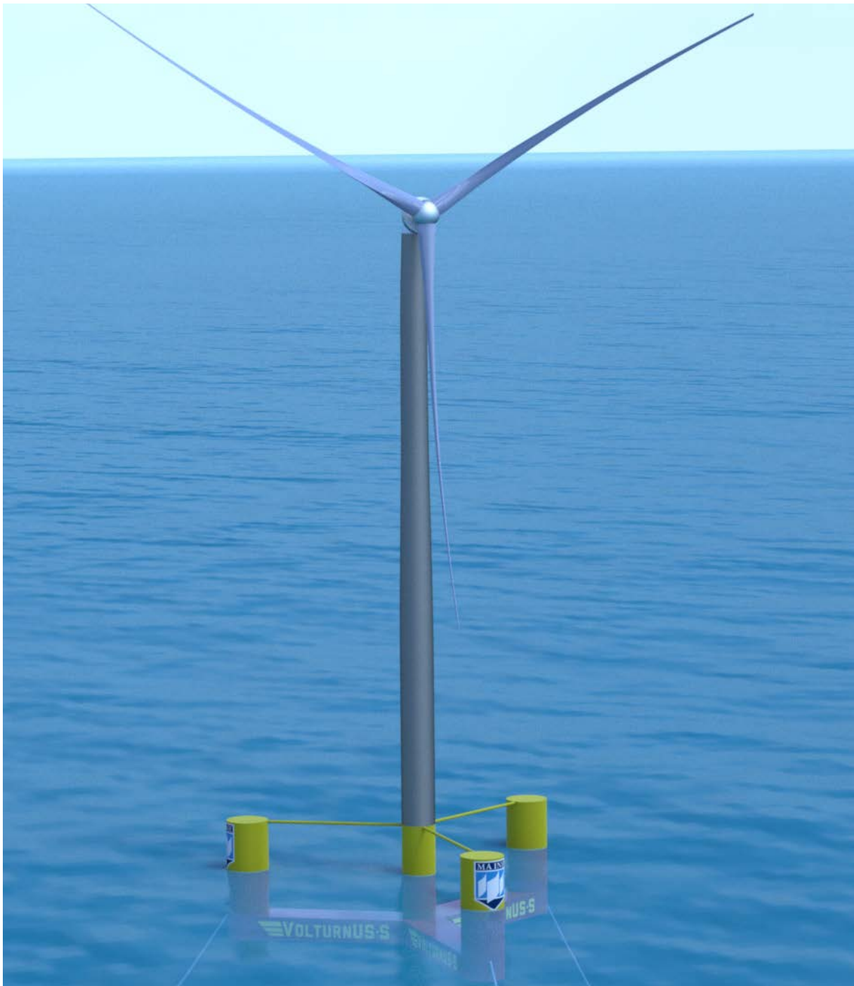
Figure 1. The UMaine VoltturnUS-S reference platform designed to support the IEA-15-240 RWT system definition. Figure courtesy of the University of Maine
