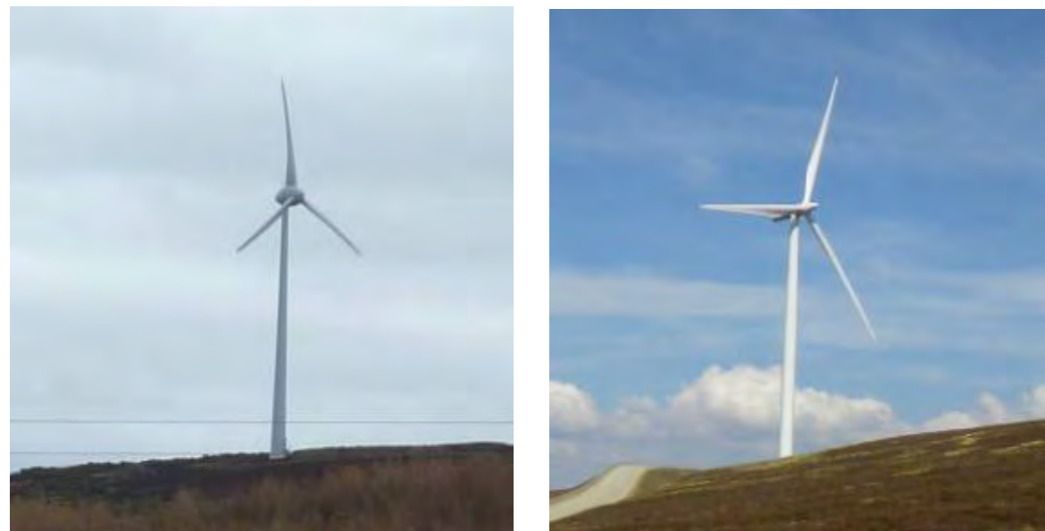
Enercon and Siemens turbines have different nacelles, blades and towers leading to significant differences in appearance
