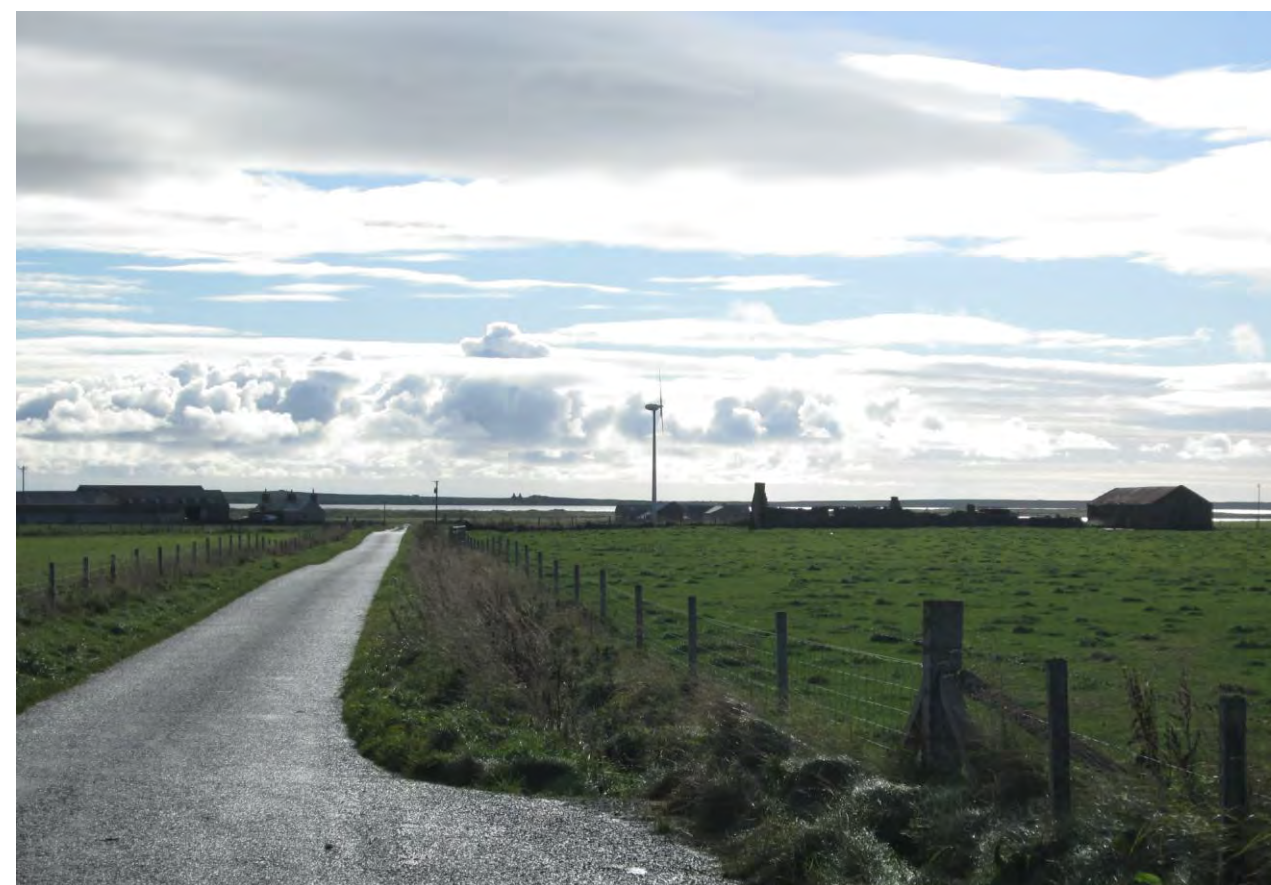
A 22m high turbine in an area of Coastal Sand Landscape. Turbines are best accommodated in the more agriculturally developed landward margins of this landscape type, such as this.
