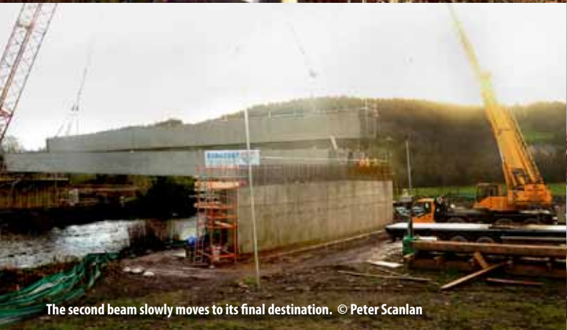
This concrete beam is now ever so slowly manoeuvred into position at the western end. © Peter Scanlan
