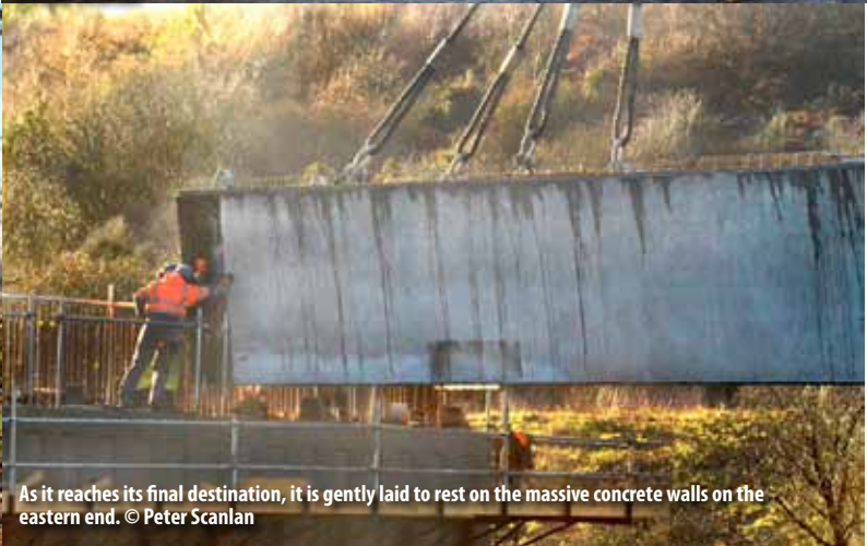
This 155 tonne, 49.9 metres concrete beam is now ever so slowly moved across the river. © Peter Scanlan
