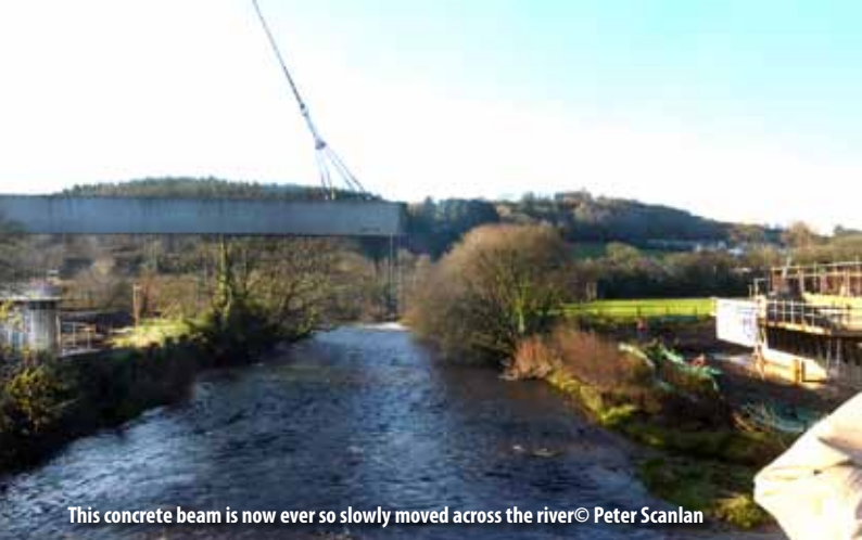
This 155 tonne, 49.9 metres concrete beam is now ever so slowly moved across the river. © Peter Scanlan
