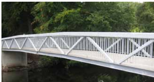
Macroom GAA Footbridge
