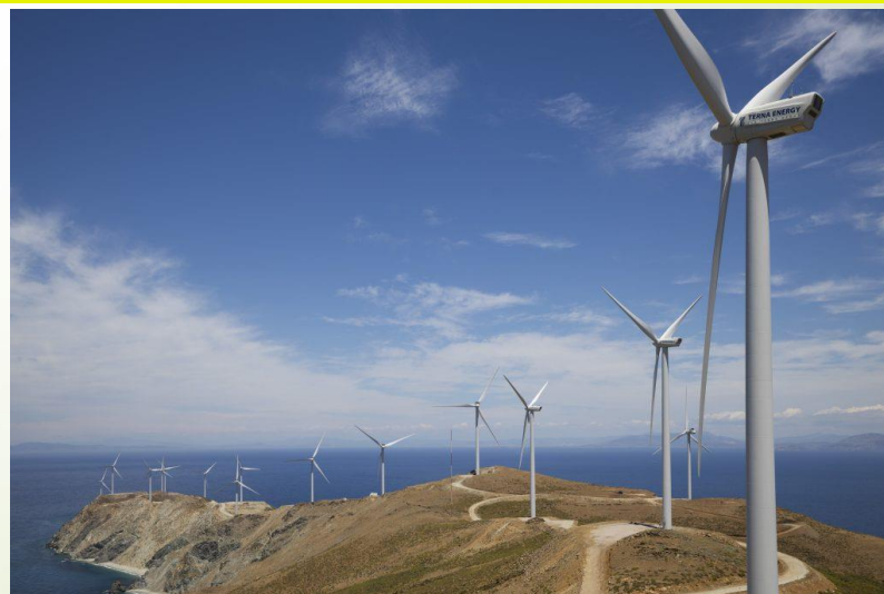
Agios Georgios island, Greece has the only onshore wind farm with offshore characteristics: submarine cables connect it to Athens' electrical grid. Photo Marios Zangas, 2016
