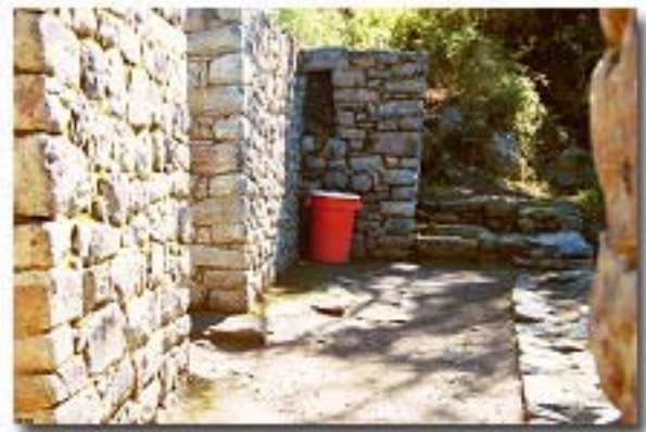
Visual impact from a garbage can in an inappropriate location
