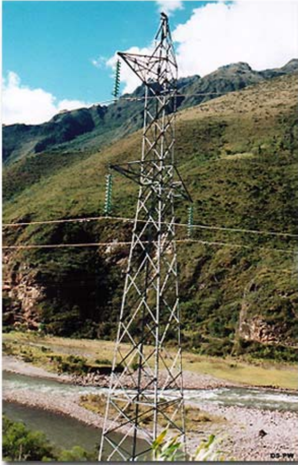
Visual impact of the transmission lines
