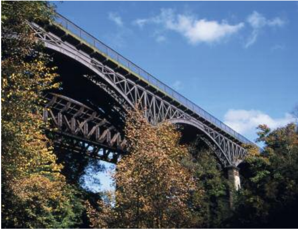
Miller's Dale viaducts
