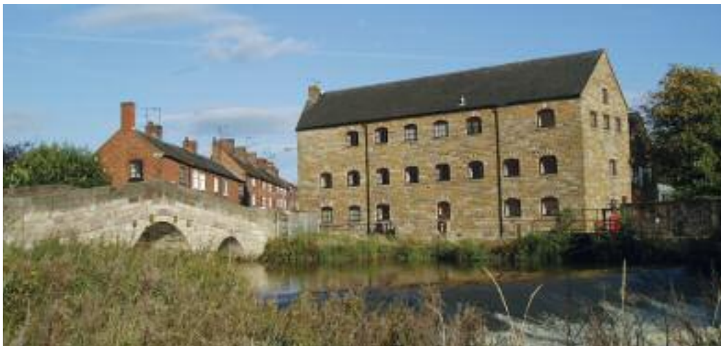
Churnet Bridge, Rocester
