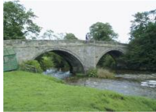
◀ Ellastone Bridge over the River Dove is on the Staffordshire - Derbyshire border
