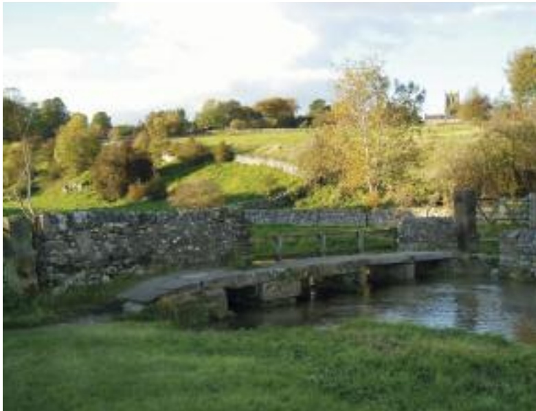
Old stone slab bridge over the River Bradford, near Youlgreave
