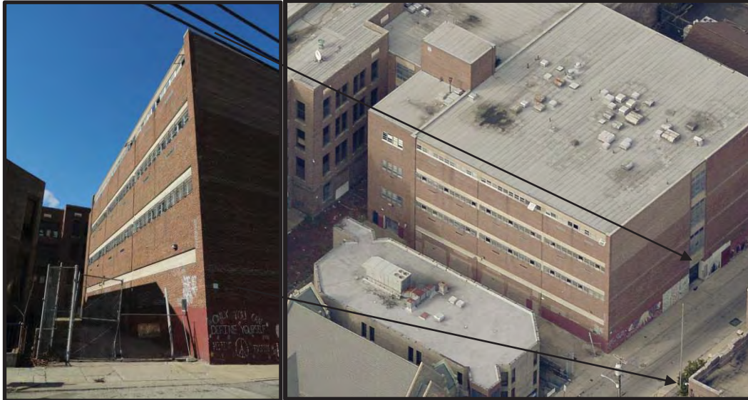
Figure 56. Left: The southwest and east elevations of the 1967–68 Addition from E. Haines Street. Source: Nicholas Covolus, 2018. Figure 57. Right: Looking north at the southwest and southeast elevations of the 1967–68 Addition. Source: Atlas, City of Philadelphia, 2018.
