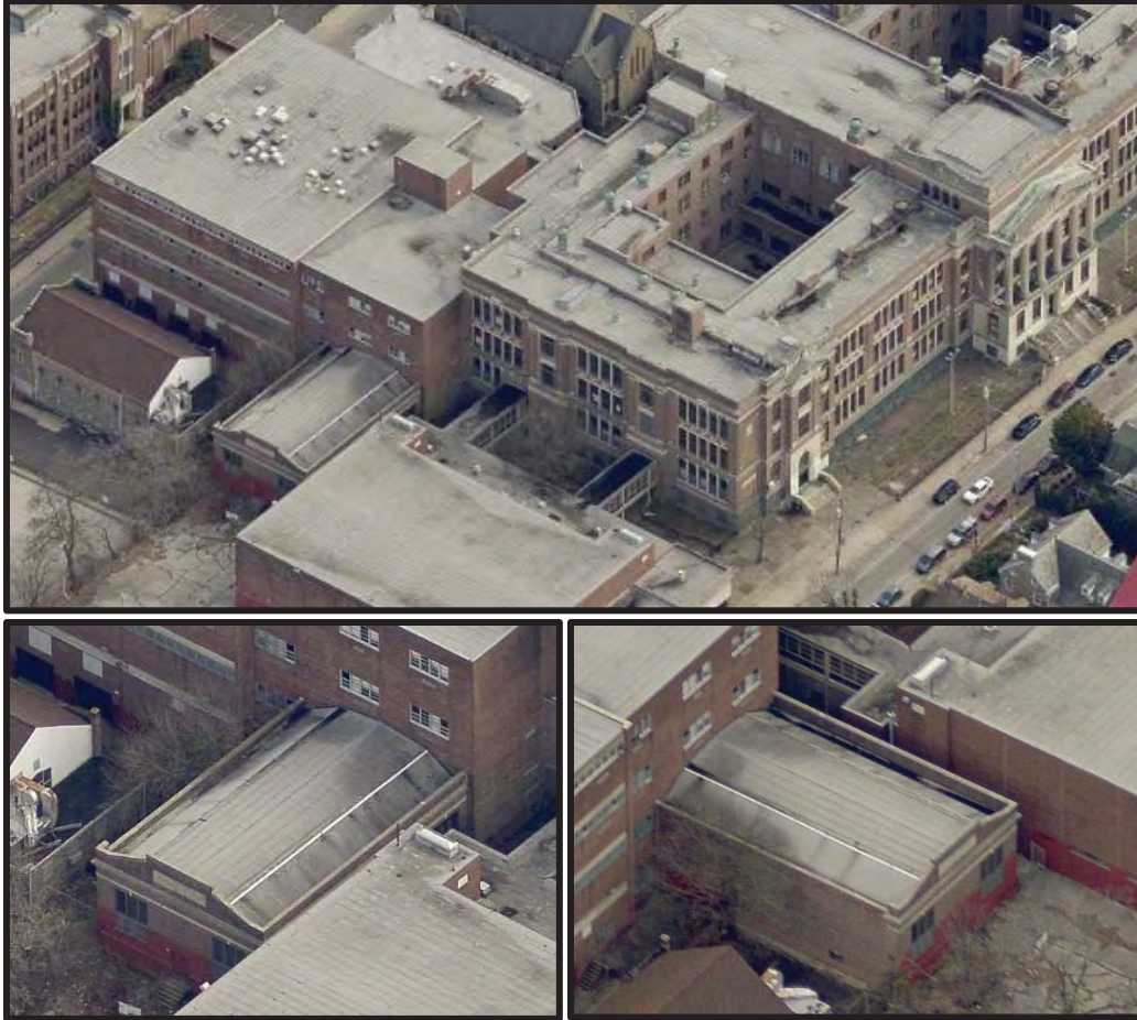
Figure 39. Top: Looking south at 1925–26 Gymnasium in the context of the Germantown High School property. Figure 40. Bottom left: Looking south at the 1925–26 Gymnasium. Figure 41. Bottom right: Looking southwest at the 1925–26 Gymnasium. Source: Atlas, City of Philadelphia, 2018.
