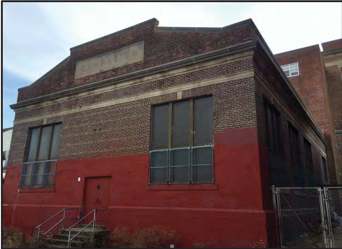
Figure 42. Top: the 1925–26 Gymnasium. Source: Photographs, Board of Education Records, CAP. Figure 43. Bottom: The northeast and northwest elevations of the 1925–26 Gymnasium. Source: Oscar Beisert, 2019.
