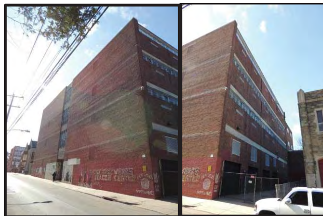
Figure 58. Left: The southeast and northeast elevations of 1967–68 Addition from E. Haines Street. Figure 59. Right: the northeast elevation of the 1967–68 Addition from E. Haines Street. Source: Nicholas Covolus, 2018.
