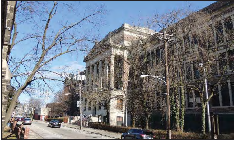
Figure 17. Looking northeast at the primary (northwest) elevation of the 1913–14 Building. Source: Nicholas Covolus, 2018.
