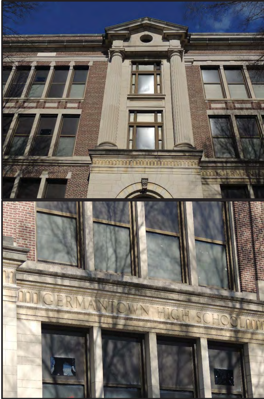
Figure 31. Top: The southwest elevation of the 1913–14 Building. Figure 32. Bottom: The southwest elevation of the 1913–14 Building. Source: Nicholas Covolus, 2018.
