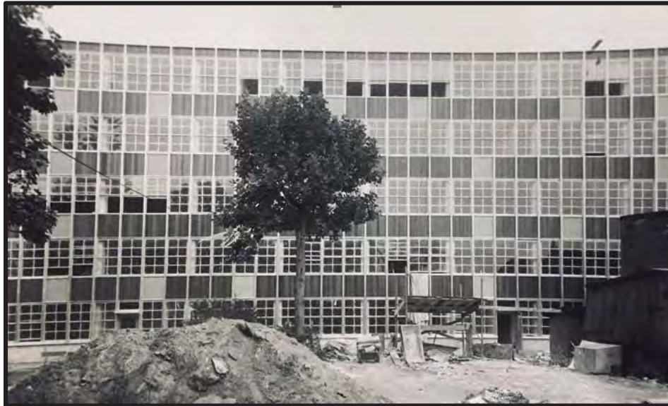
Figure 124. The southwest elevation of the 1964–65 Gymnasium. Source: Photographs, Board of Education Records, CAP.
