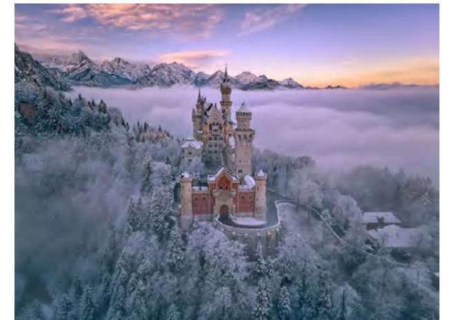
Judith Kuhn - Snow and Fog in Wonderland 1st Place in Architecture, Historic
