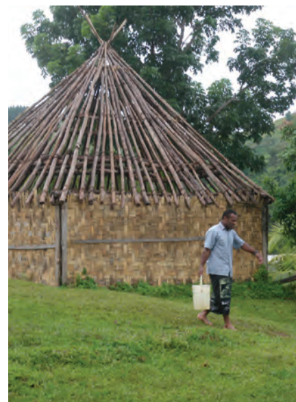
Woven thatch of Schizostachyum glaucifolium for walls of traditional Fijian Bure, Nausori Highlands, Fiji (image: Lex Thomson).
