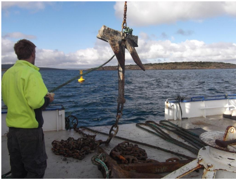
Figure 29. Anchors used for securing horizontal 35mm rope
