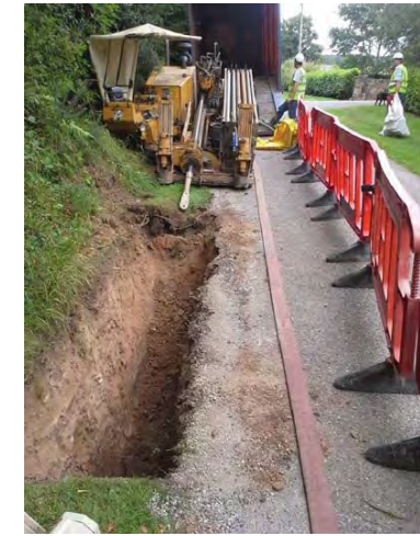
Typical Drilling Rig and Launch Pit
