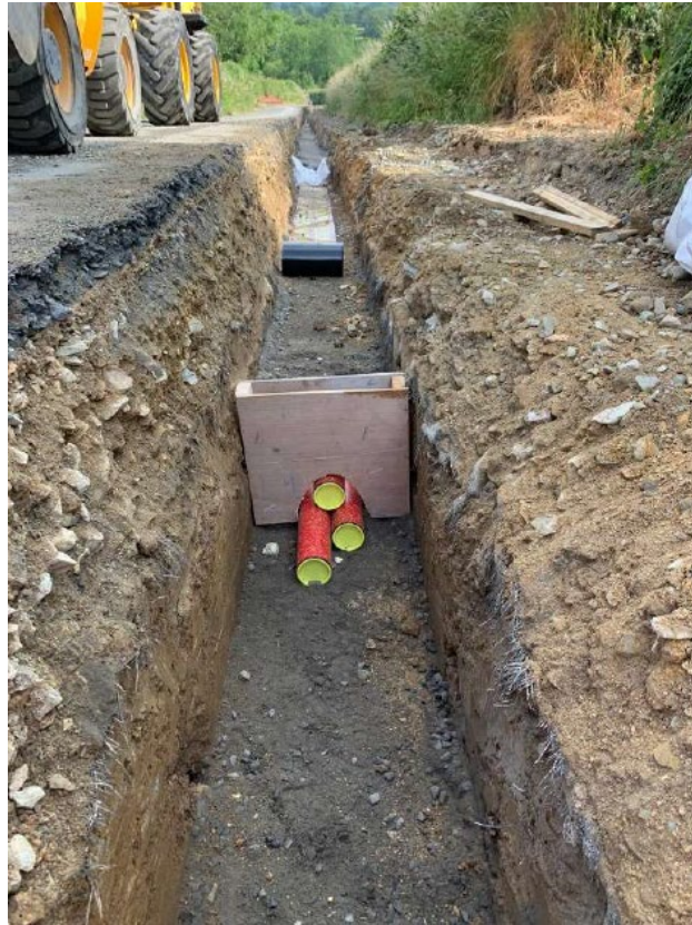
Figure 3-4: Typical 38kV Underground Duct Installation
