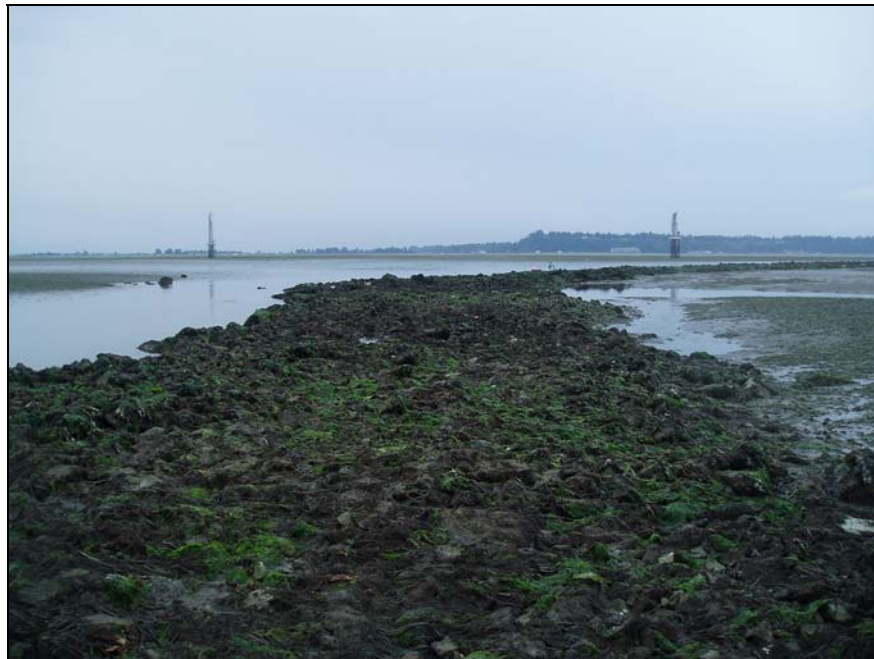
Photo 3: Crest Protection Monitoring XS 3 looking northeast, July 2008
