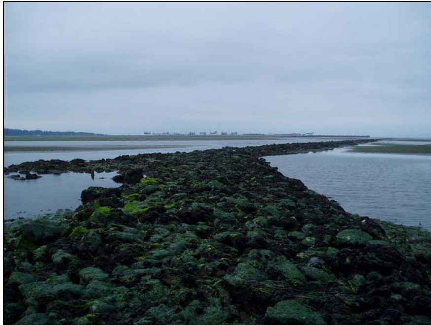
Photo 5: Crest Protection Monitoring XS 5 looking southeast, July 2008
