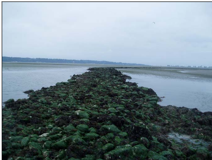
Photo 4: Crest Protection Monitoring XS 4 looking east, July 2008
