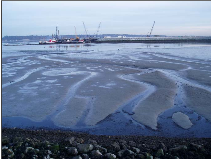
Photo 7: New drainage channels looking towards the East
