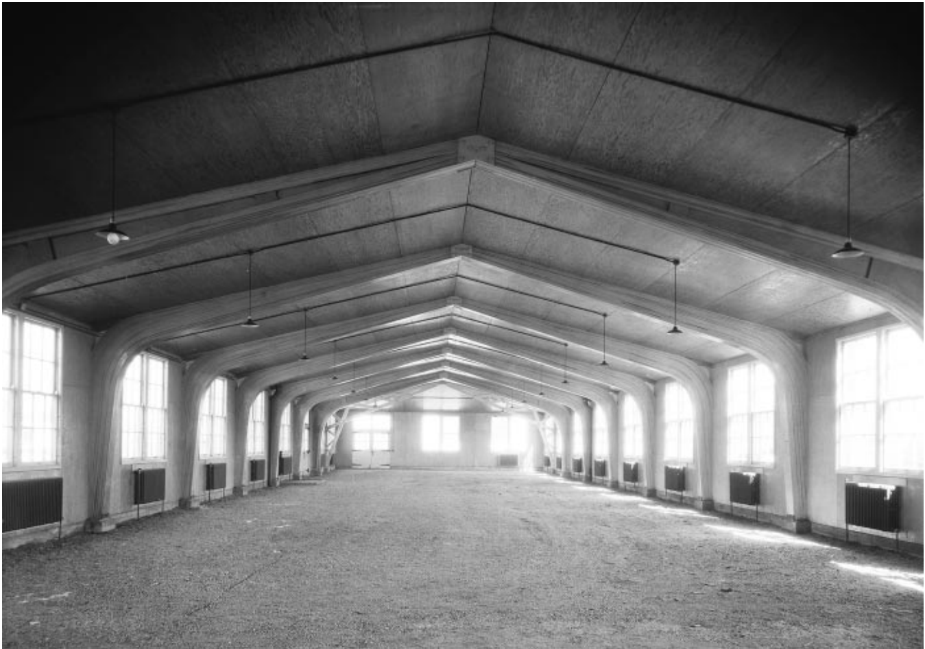
Figure 11–3. Erected in 1934 at the Forest Products Laboratory in Madison, Wisconsin, this building is one of the first constructed with glued-laminated timbers arched, designed, and built using engineering principles.
