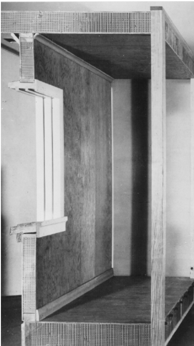
Figure 11–13. Cutaway to show details of sandwich construction in an experimental structure.
